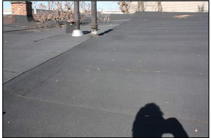
2. Modified bitumen membrane
