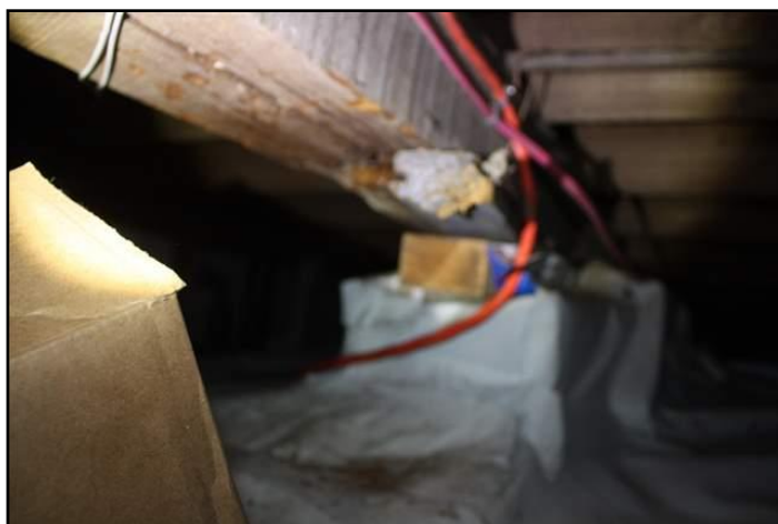
13. Weak connection to column
