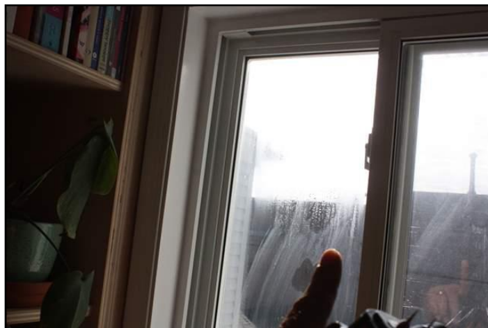
25. Lost seal on double or triple glazing
