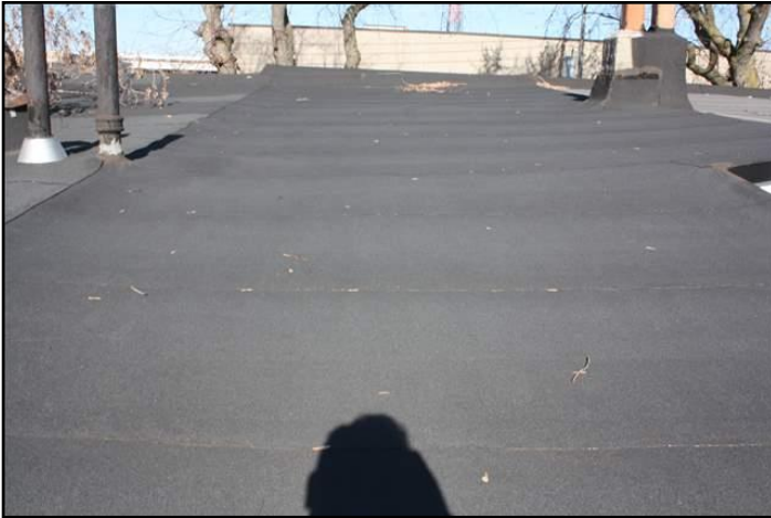
1. Modified bitumen membrane
