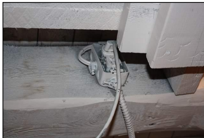
19. For outlet (receptacle) is missing
