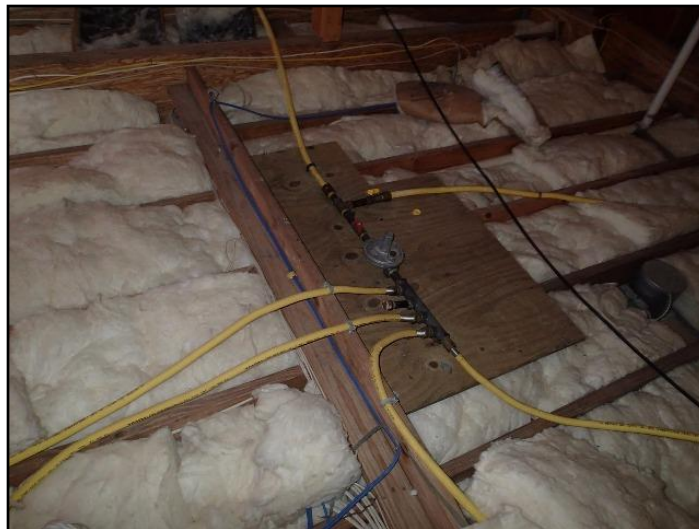
40. CSST (Corrugated Stainless Steel Tubing)
