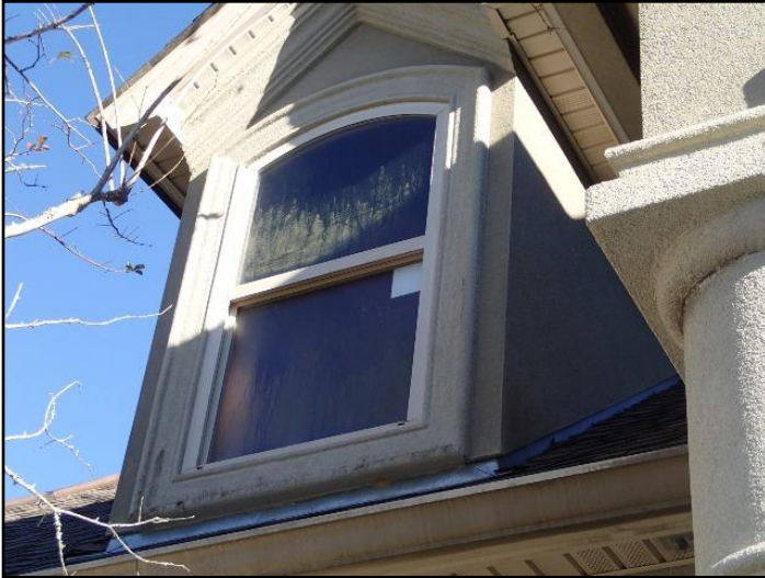
51. Lost seal on double or triple glazing
