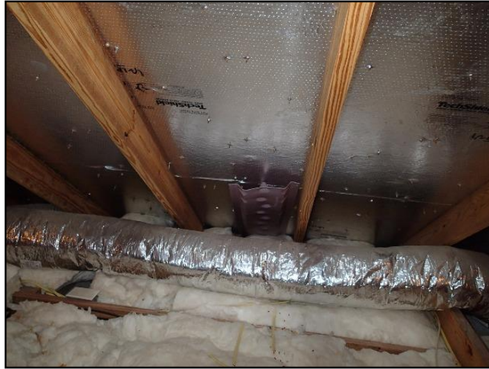
34. Baffles installed at rafter openings.
