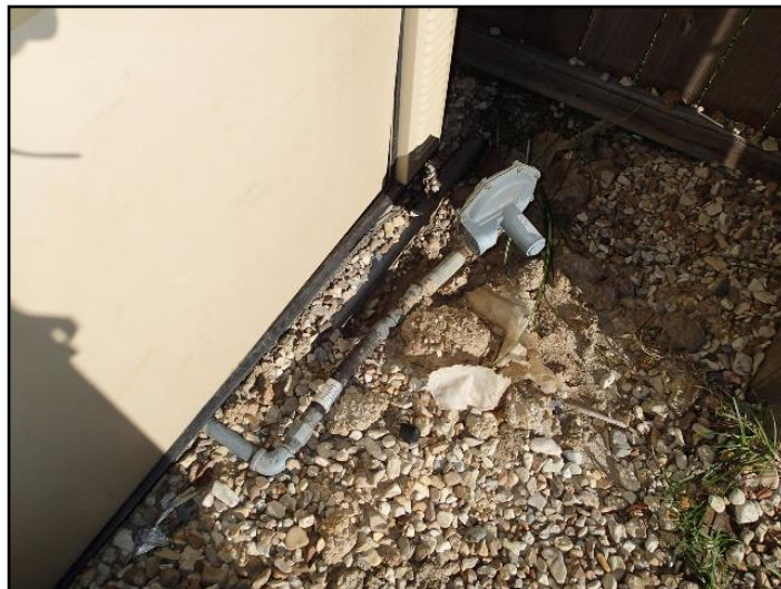
42. Missing shut off valve
