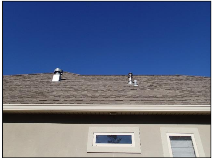
2. Asphalt shingles
