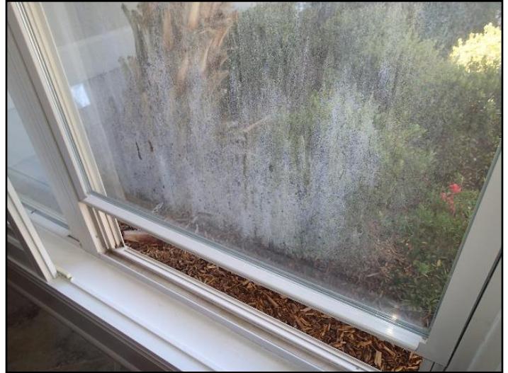
52. Lost seal on double or triple glazing
