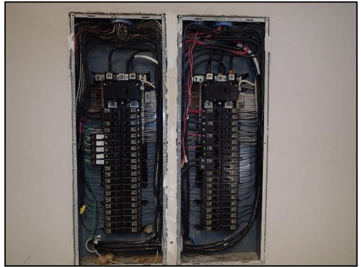
17. Electrical panels with cover removed.
