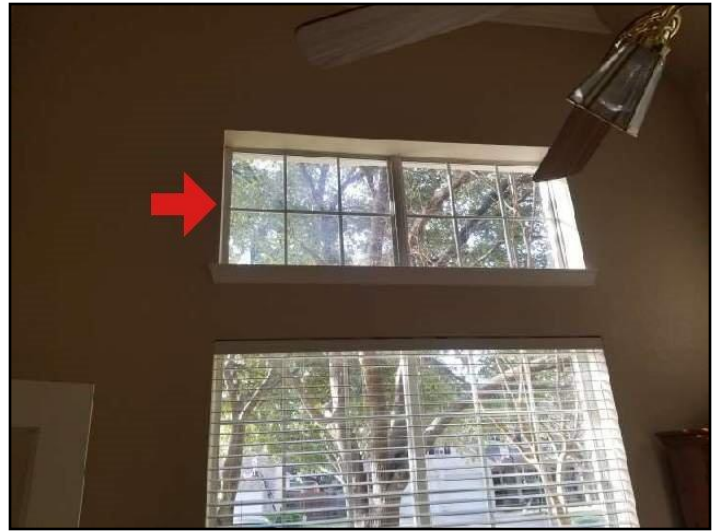
38. Lost seal on double or triple glazing
