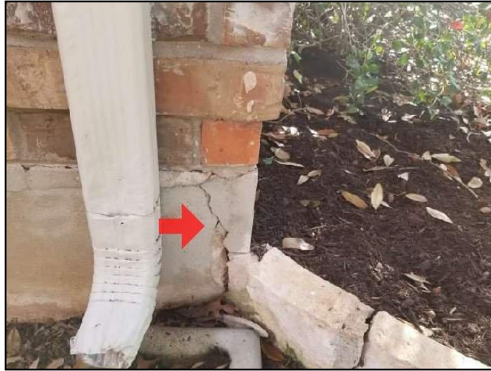
14. Corner cracks observed at the corners of th...
