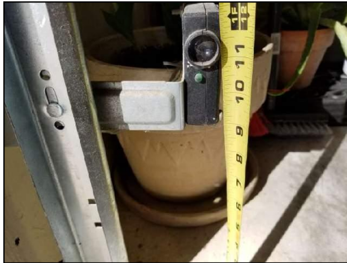
40. Sensors poorly located
