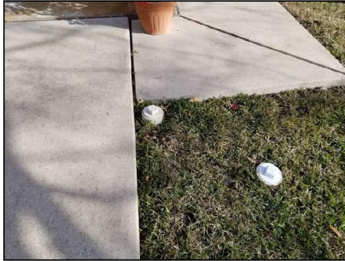
33. Main Drain Cleanout Location:
