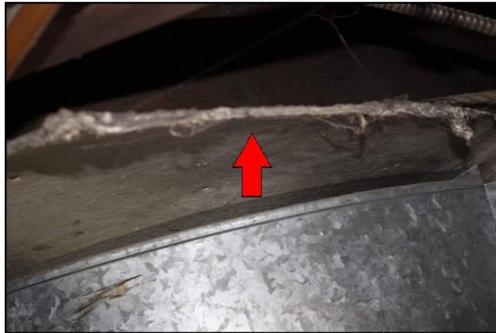
23. Possible asbestos containing materials
