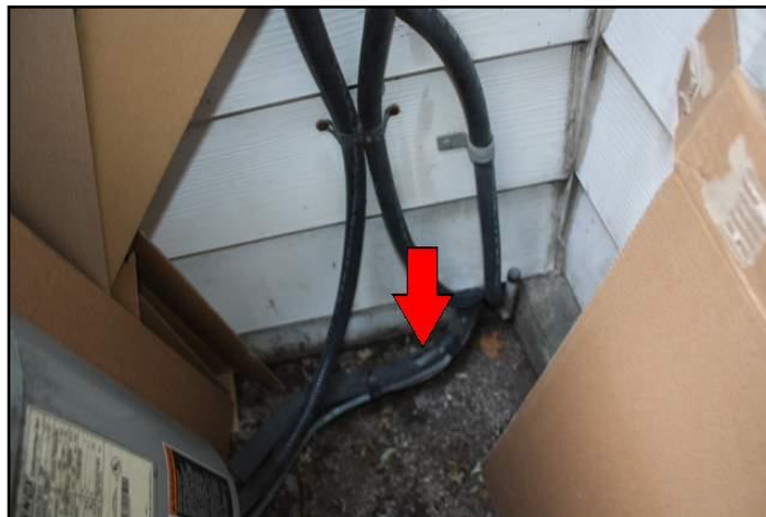
21. Insulation - missing
