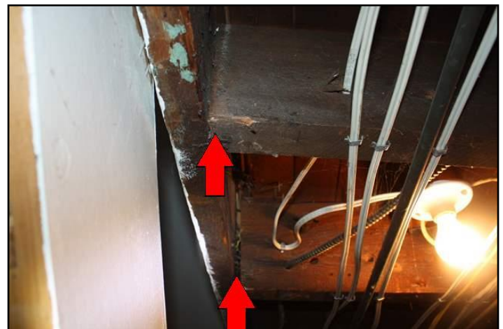
13. Poor end bearing, joist hanger connections
