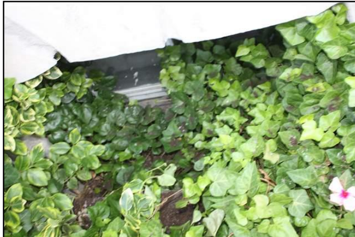
10. Window sill is at or below grade.
