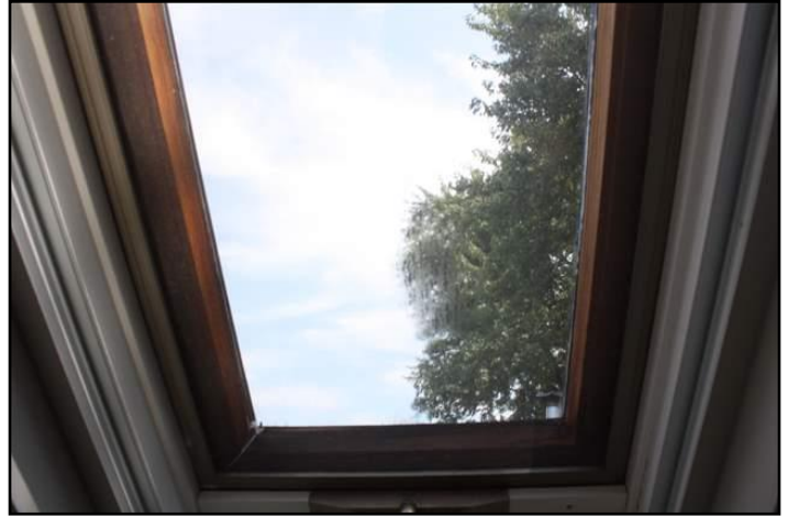
9. Lost seal on double or triple glazing
