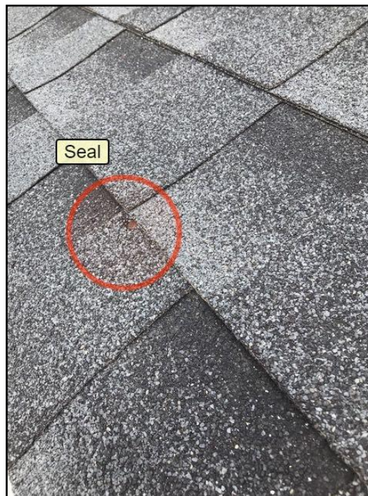
Exposed fasteners
