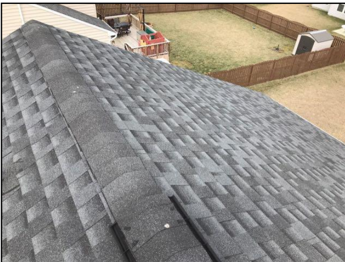
Asphalt shingles
