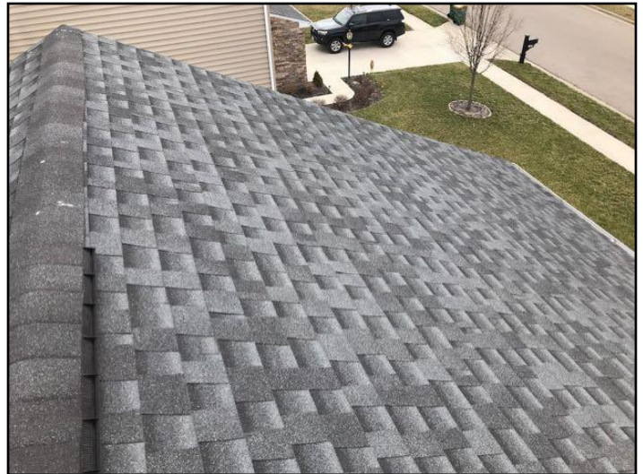
Asphalt shingles
