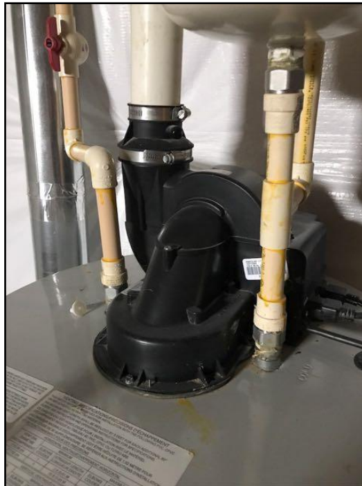
Direct vent - sealed combustion
