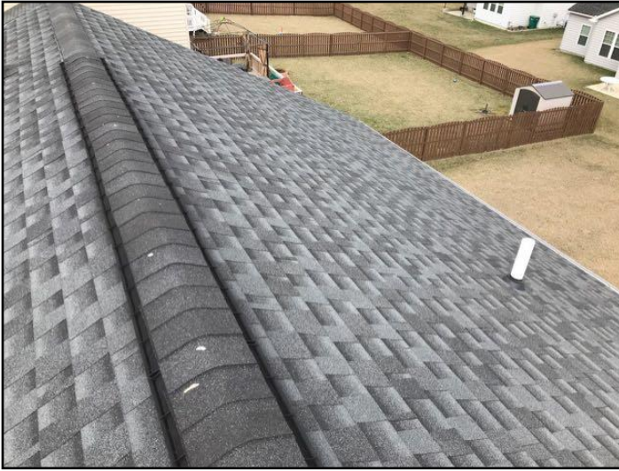
Asphalt shingles
