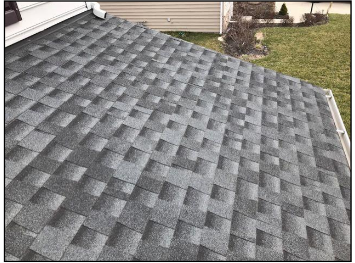
Asphalt shingles
