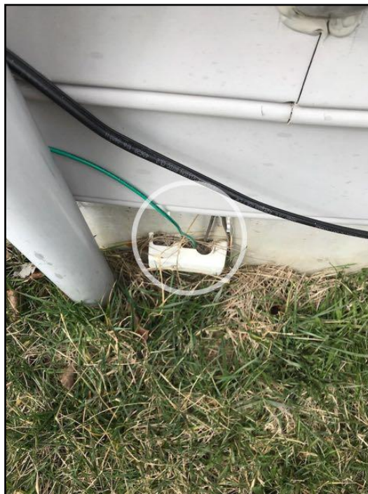
Copper - ground rods
