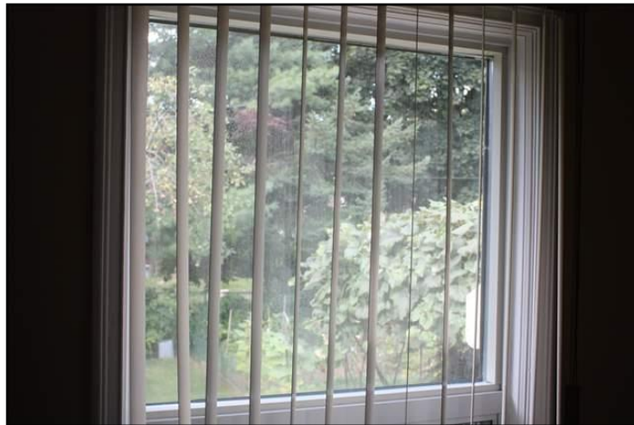
4. Lost seal on double or triple glazing
