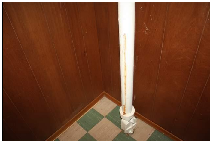
21. The cast iron waste piping is near the end...
