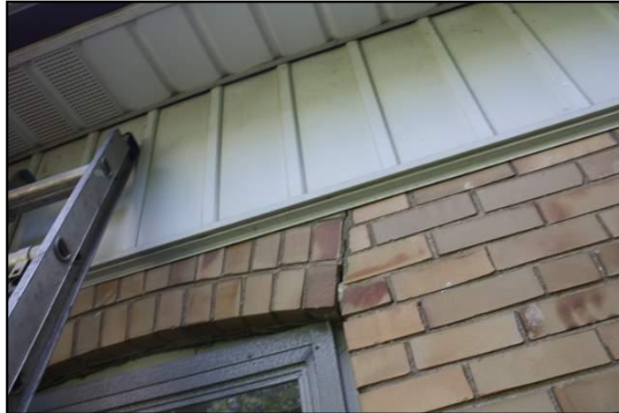
9. Mortar deteriorated
