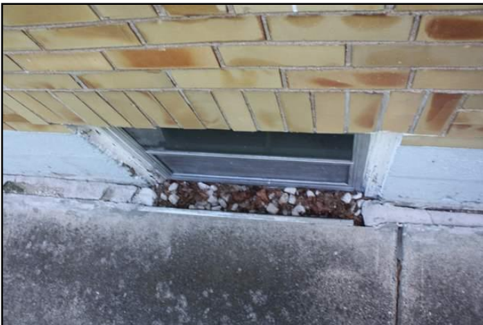
5. Window sill is at or below grade.
