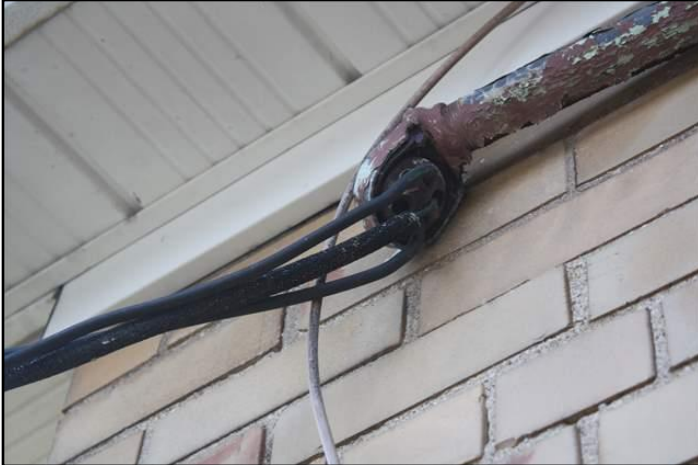
12. Inadequate service size
