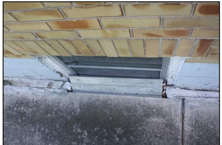
6. Window sill is at or below grade.
