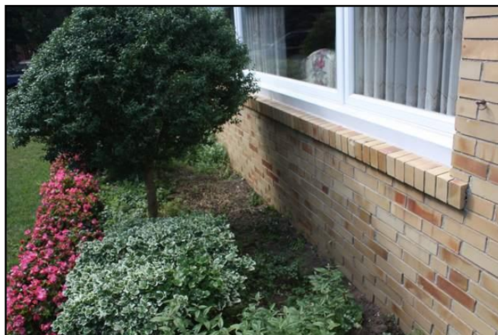
8. Masonry too close to grade
