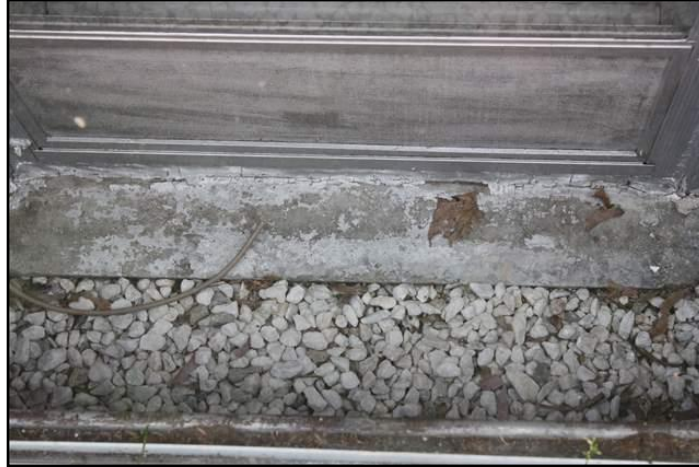
7. Window sill is at or below grade.
