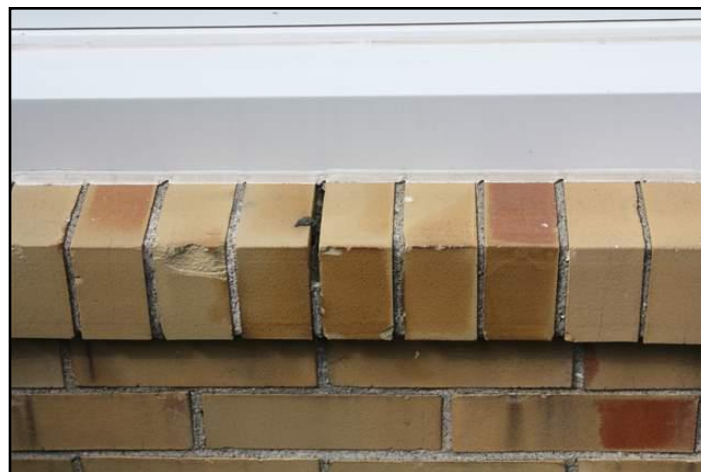
3. Mortar deterioration
