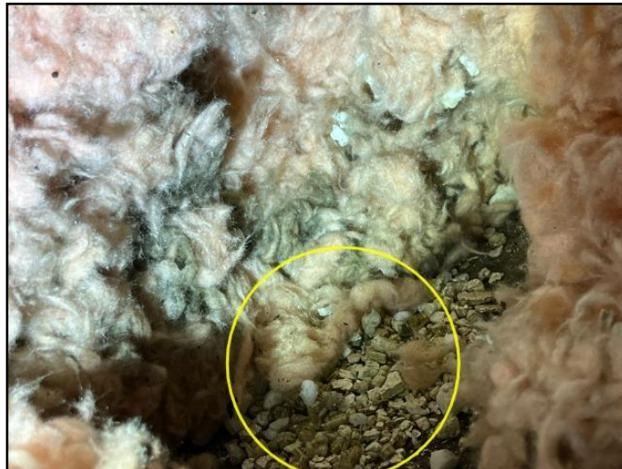
6. vermiculite insulation
