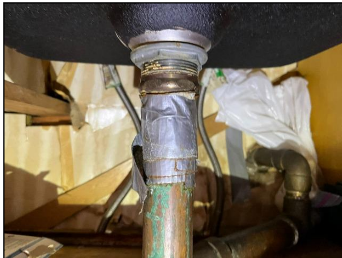
9. Nonstandard materials and patches
