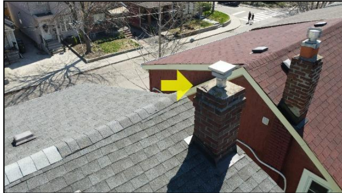
5. No drip edge on cap (crown)
