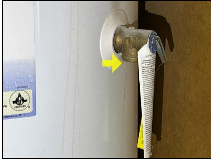
8. Discharge tube missing
