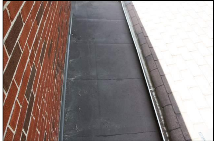
2. Modified bitumen membrane
