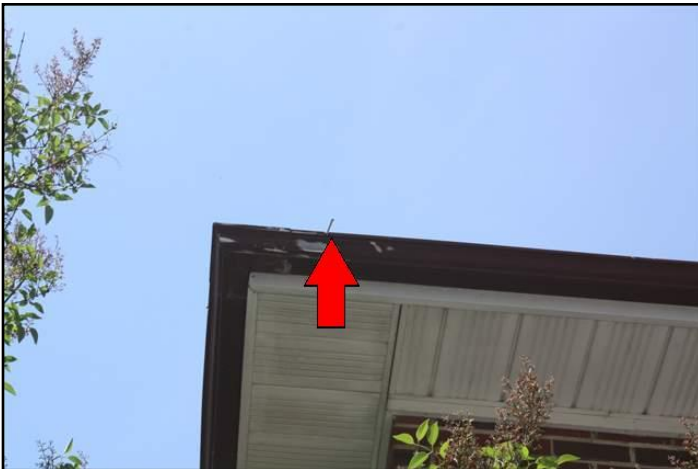
9. Aging - Wear and tear noted. Fasteners...
