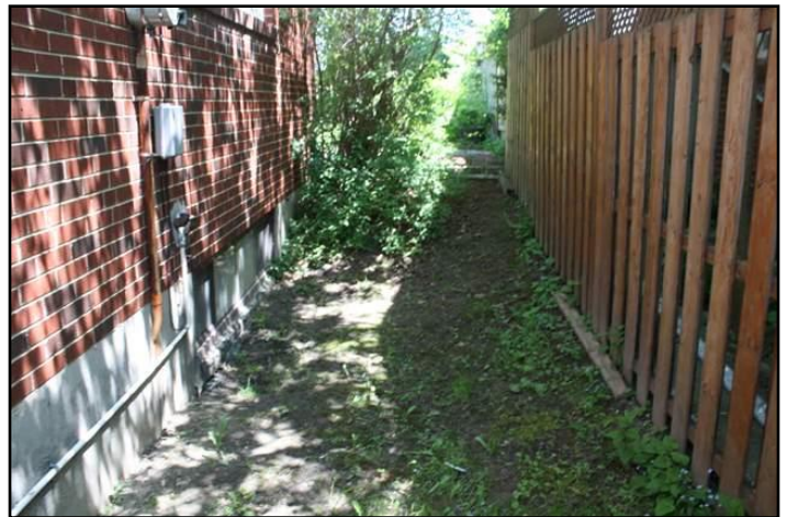
24. Improper slope or drainage
