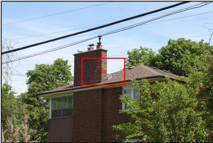
36. Loose, missing or deteriorated mortar
