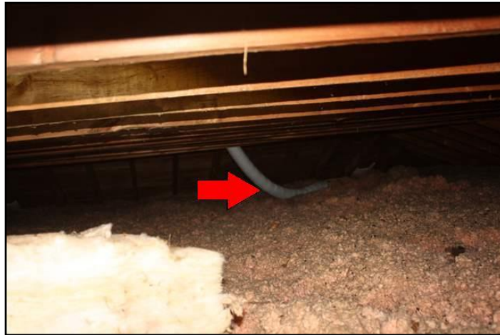
44. Not insulated in unconditioned space
