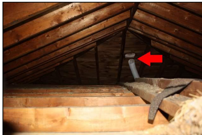
45. Poor termination location
