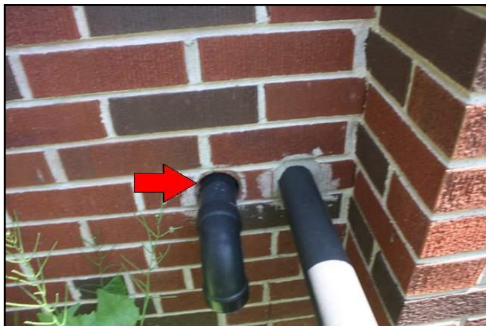
12. Caulking missing or ineffective
