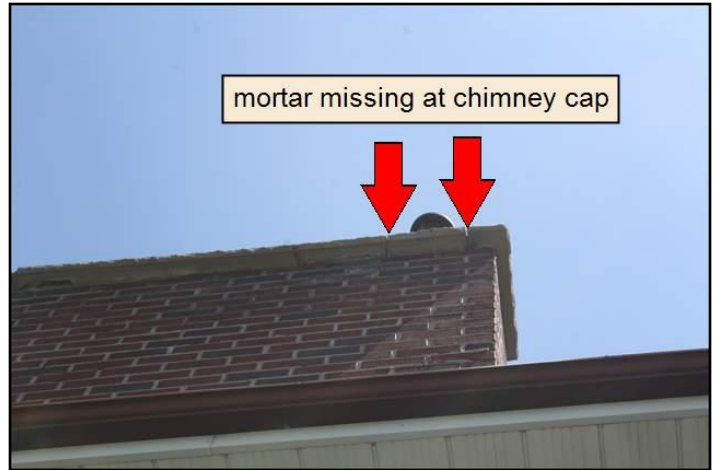
37. Loose, missing or deteriorated mortar
