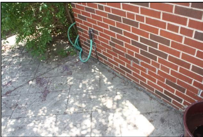
31. Masonry too close to grade
