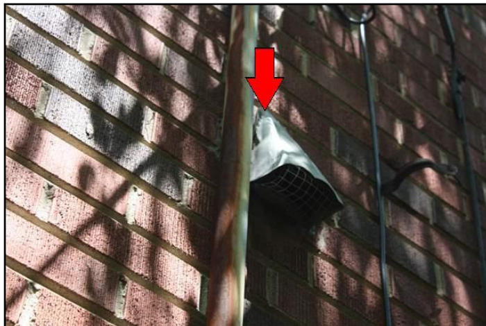
11. Caulking missing or ineffective
