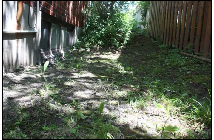
22. Improper slope or drainage
