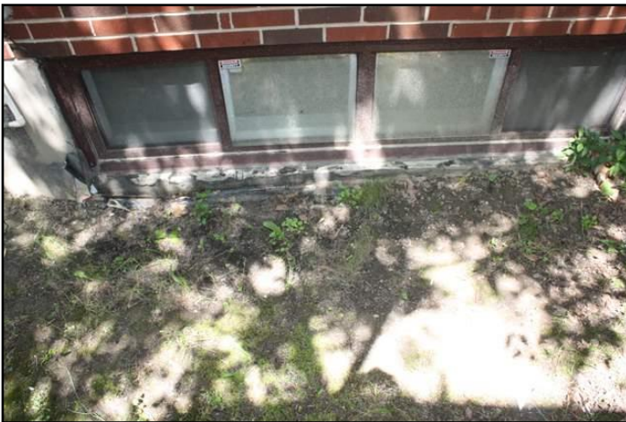
23. Improper slope or drainage
