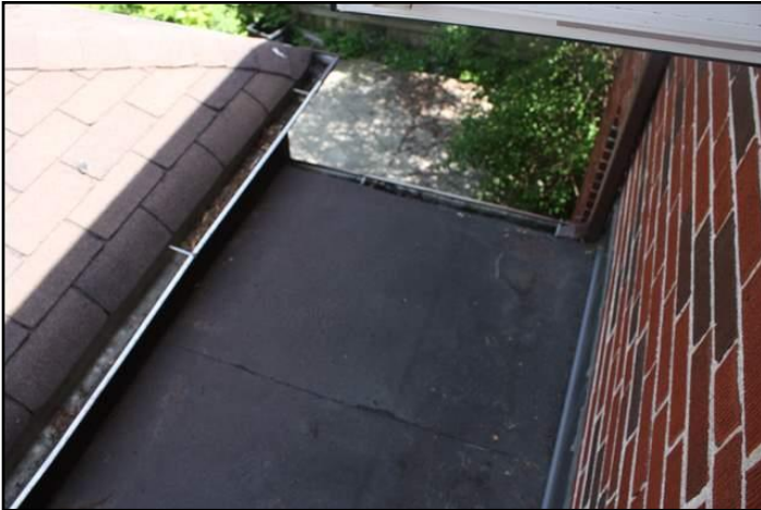
1. Modified bitumen membrane
