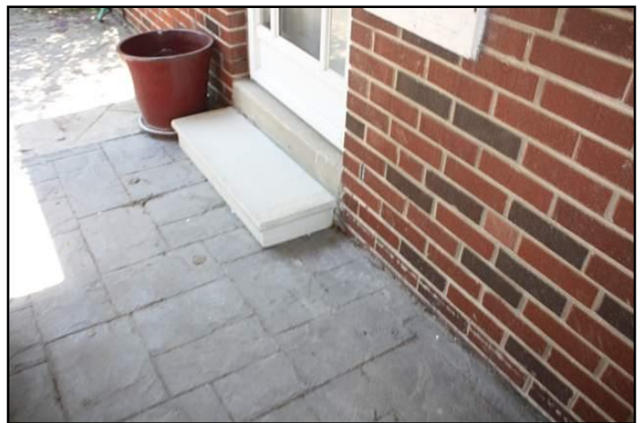
32. Masonry too close to grade
