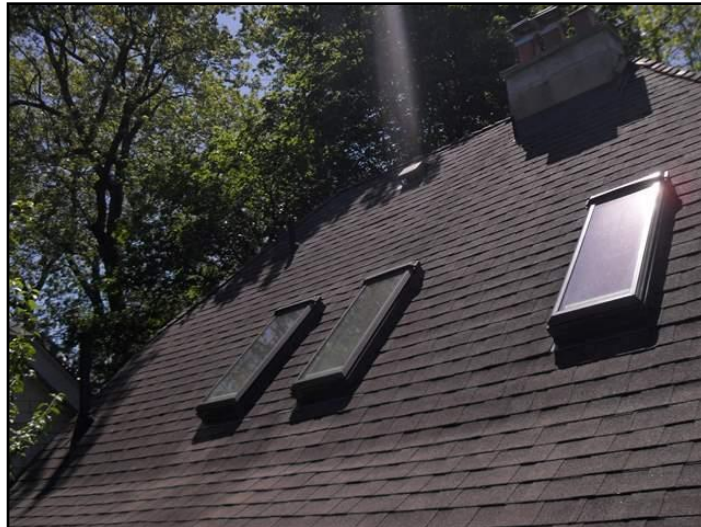
Skylight(s) - vulnerable area -
