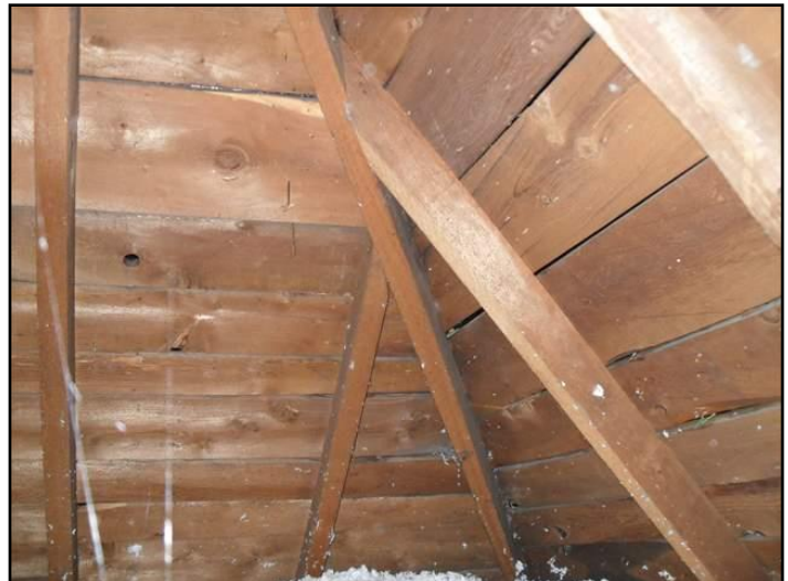
Rafters/roof joists
