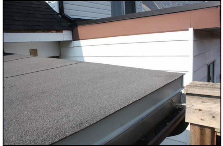
2. Modified bitumen membrane
