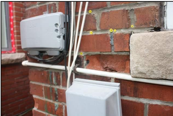
9. Spalling
