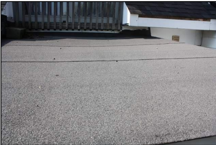
3. Modified bitumen membrane
