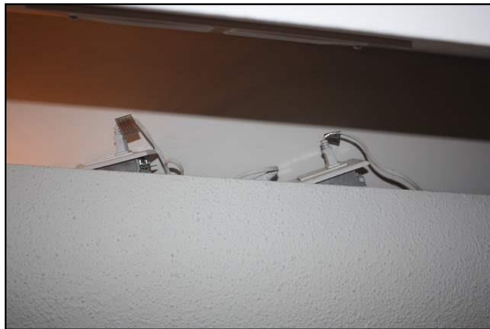
30. Outlets not well secured
