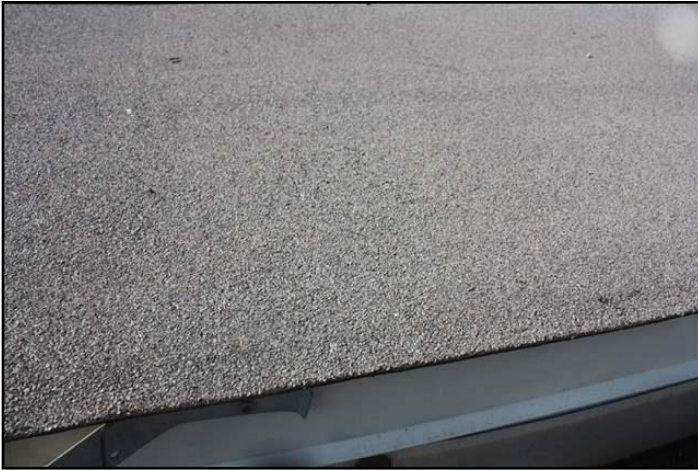
1. Modified bitumen membrane
