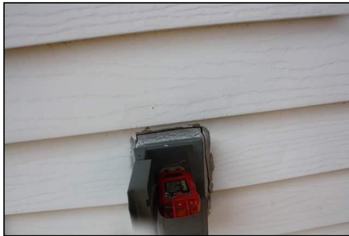
31. GFCI/GFI needed (Ground Fault Circuit...
