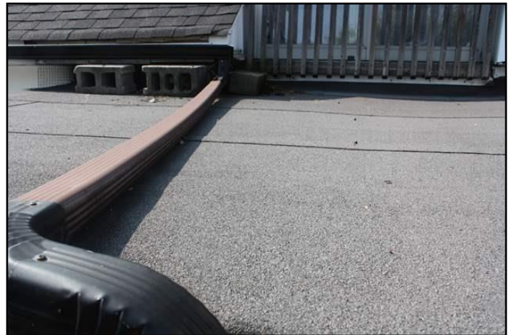
4. Modified bitumen membrane
