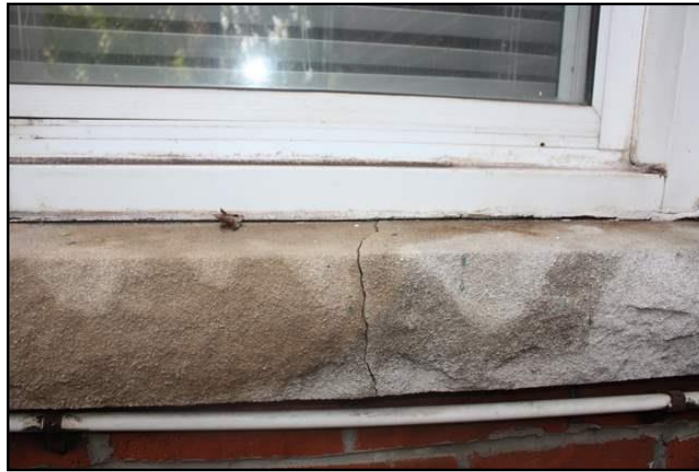
11. Sill deteriorated
