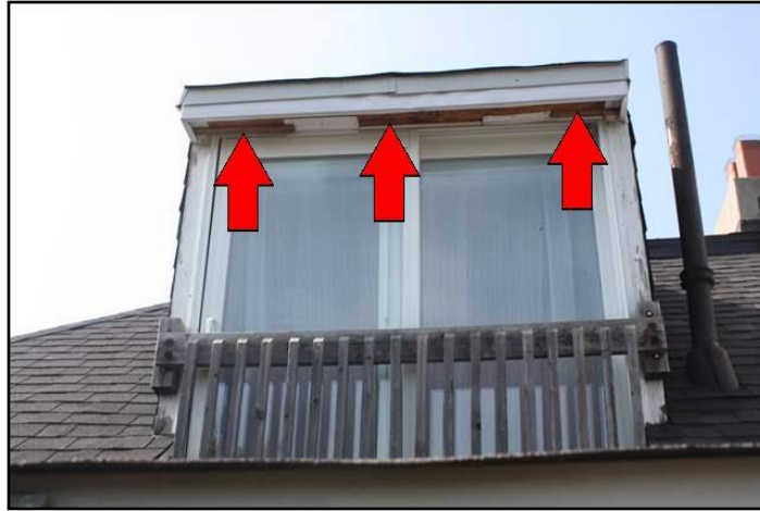
6. Flashings incomplete or ineffective
