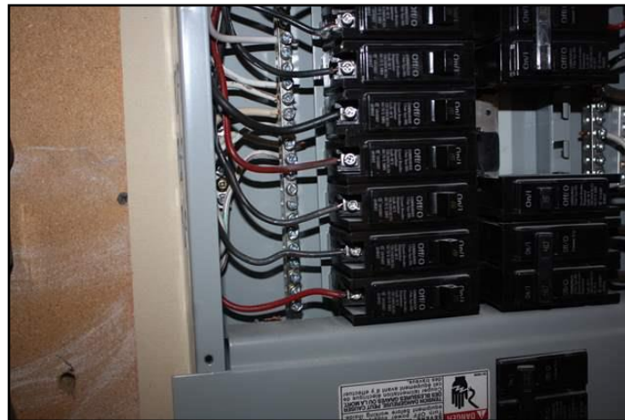
24. No links for multi-wire circuits
