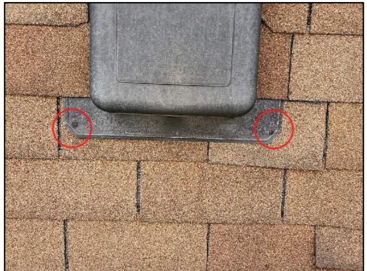
Exposed fasteners not sealed
