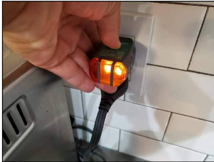
GFCI/GFI needed (Ground Fault Circuit...
