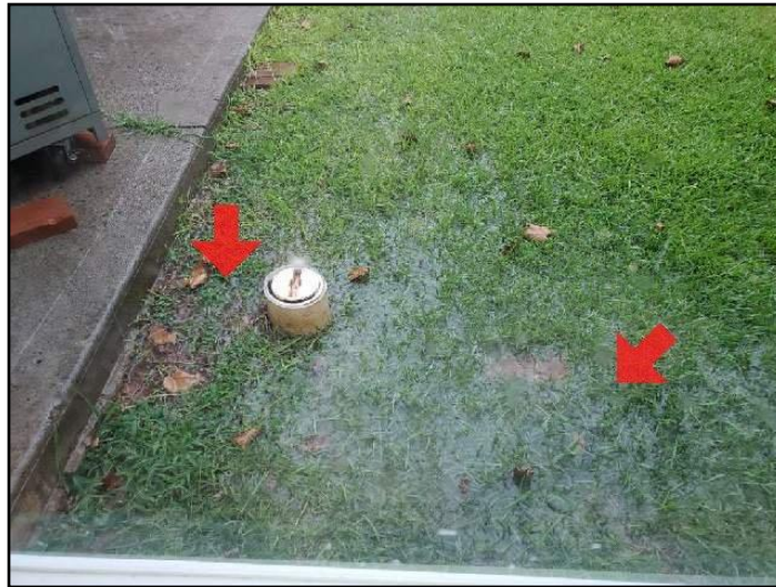
Improper slope or drainage
