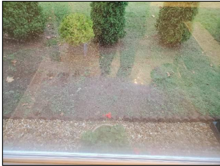
Lost seal on double or triple glazing
