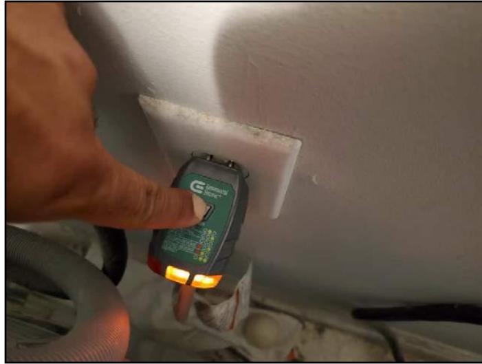
GFCI/GFI needed (Ground Fault Circuit...
