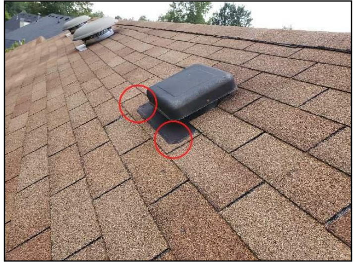
Exposed fasteners not sealed
