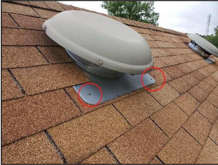
Exposed fasteners not sealed
