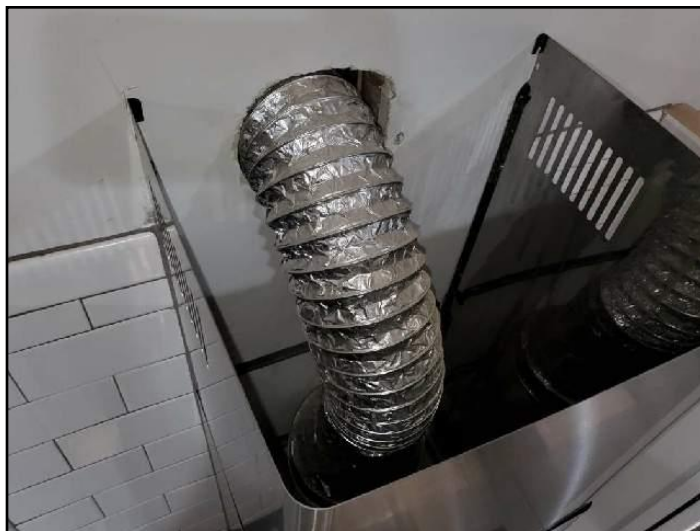
Venting arrangement poor
