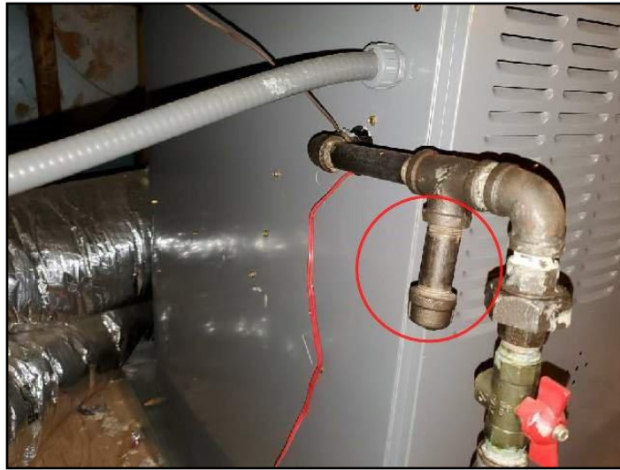
Improper sediment trap
