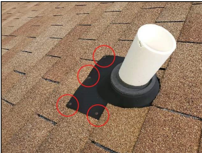
Exposed fasteners not sealed
