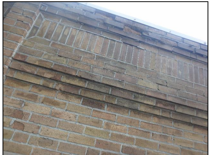
3. Spalling
