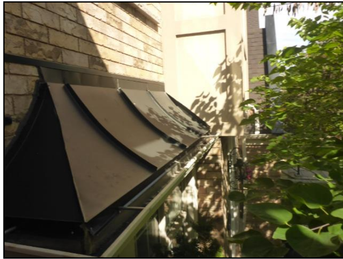
Metal roof at front bay
