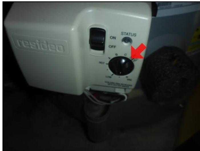
Thermostat at tank set very high
