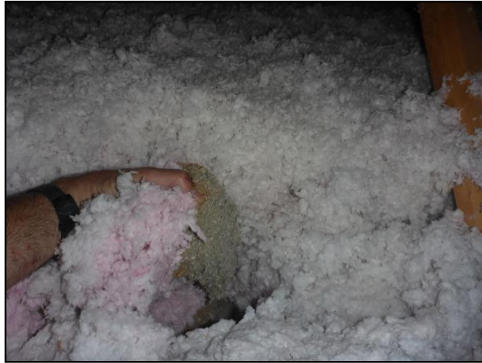
Base layer of cellulose insulation noted
