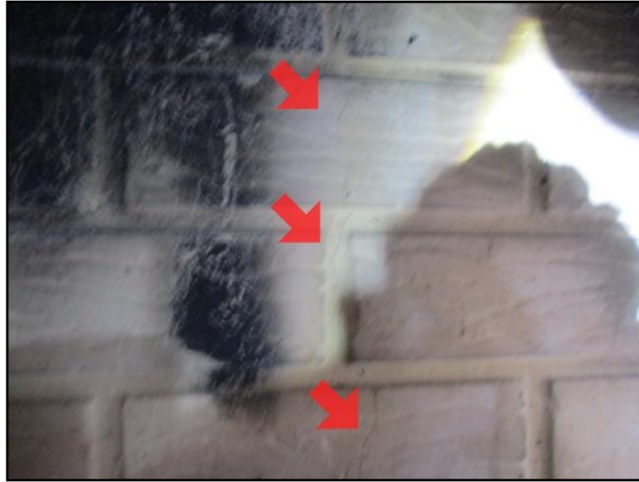
Cracked masonry or refractory
