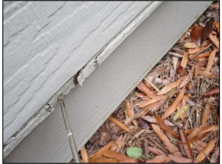
Rot or insect damage
