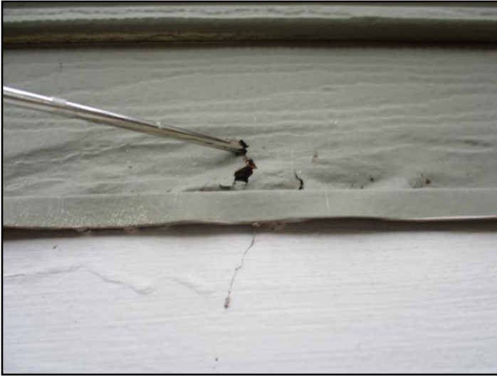
Rot or insect damage
