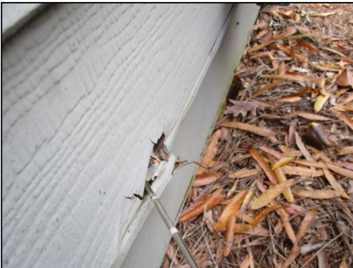
Rot or insect damage
