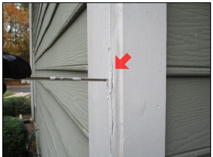
Rot or insect damage
