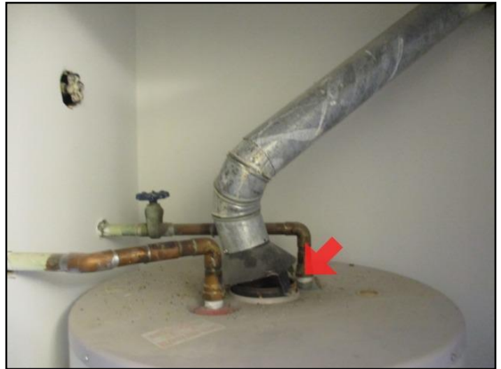
Spillage or backdraft at the draft hood
