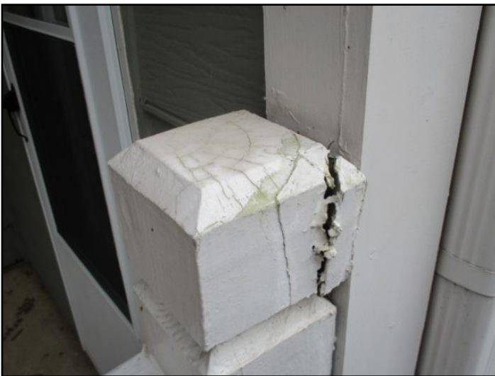
Rot or insect damage
