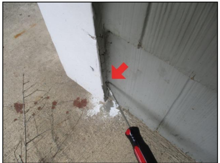
Rot or insect damage
