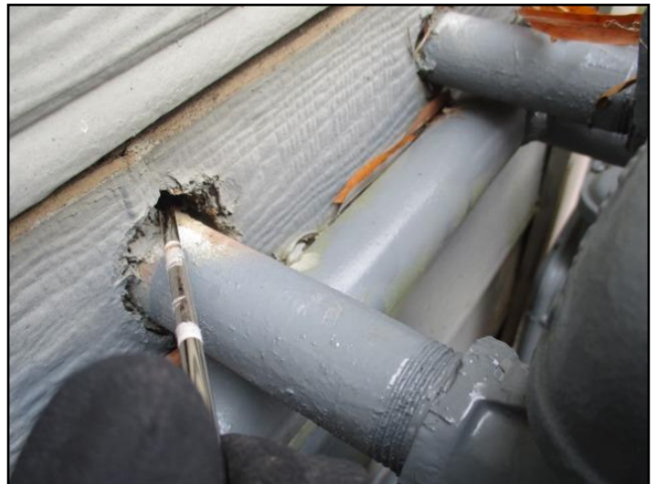
Rot or insect damage
