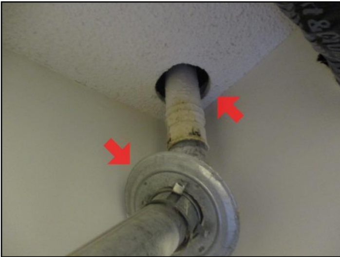
Spillage or backdraft at the draft hood
