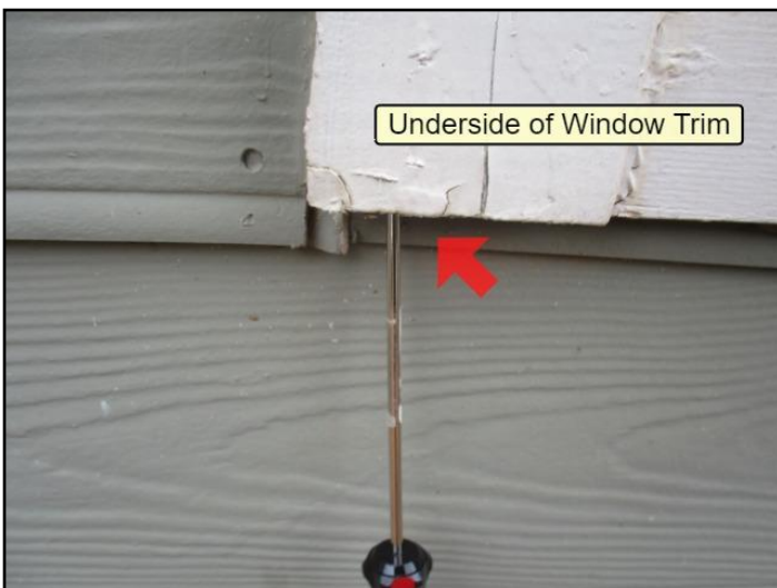
Rot or insect damage
