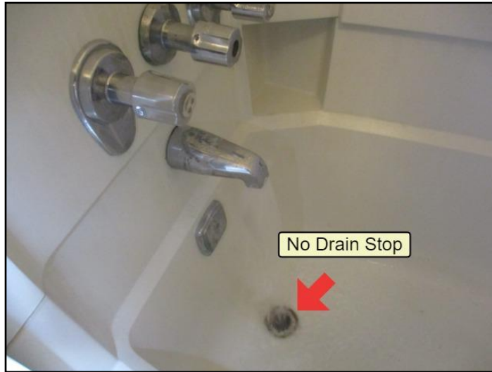
Drain stop missing
