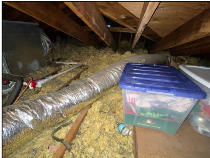
Blown loose fill insulation
