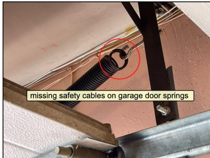
Missing safety cables through extension...
