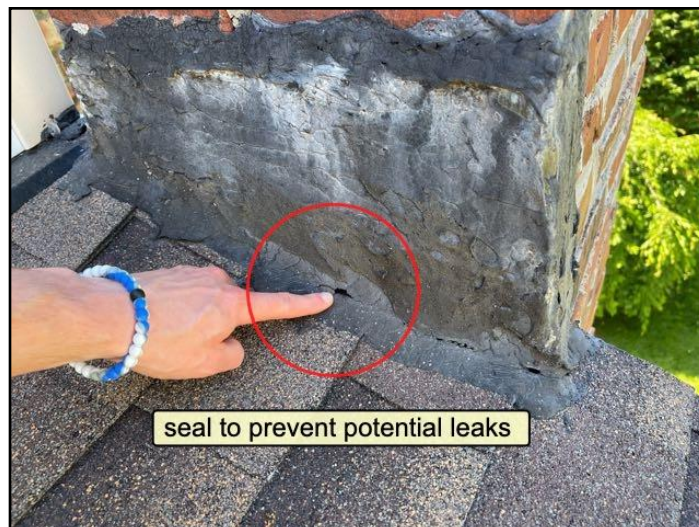
Damage, loose, open seams, patched
