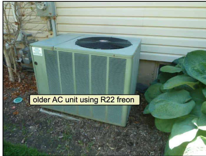
AC is old using R-22 freon in system. This...
