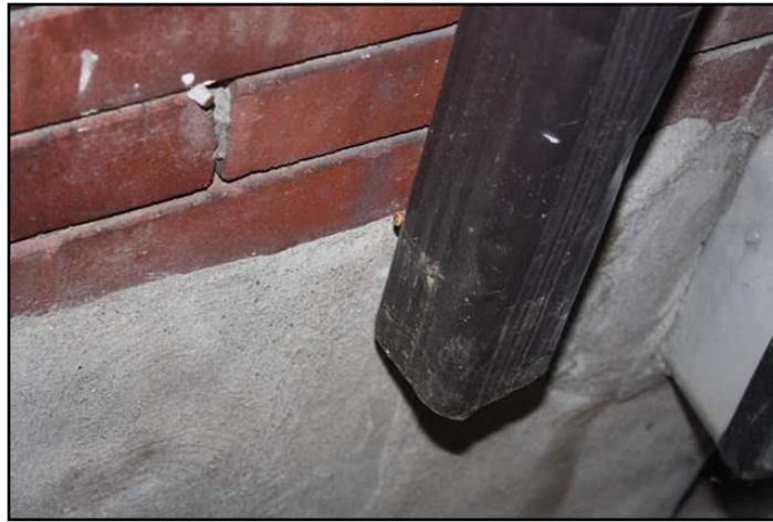
4. Should discharge 6 feet from building
