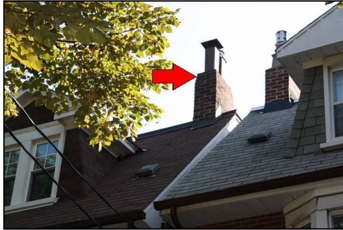
14. Missing Chimney Cap
