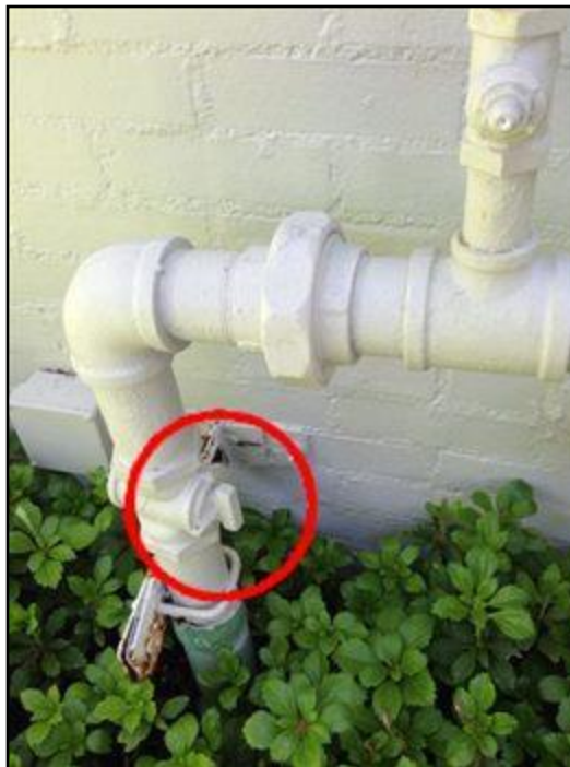
Exterior wall/main gas shutoff
