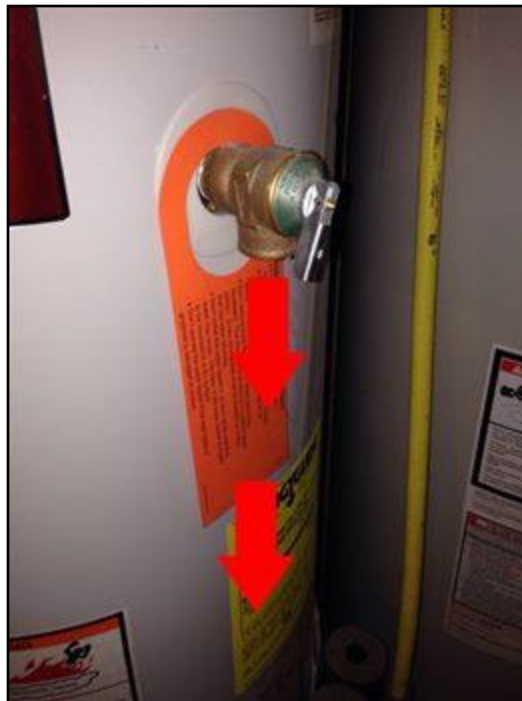
Discharge tube missing
