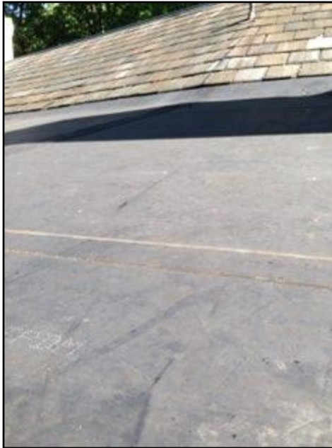
Rubber based roofing material
