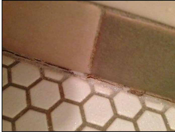
Caulking loose, missing or deteriorated
