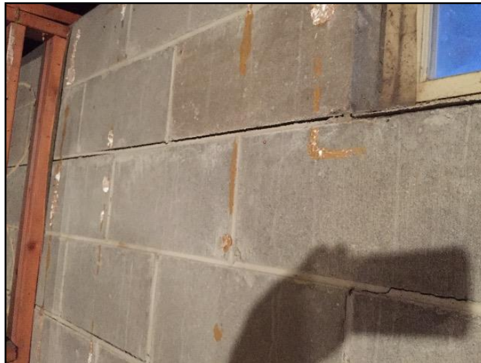
Cracked horizontally
