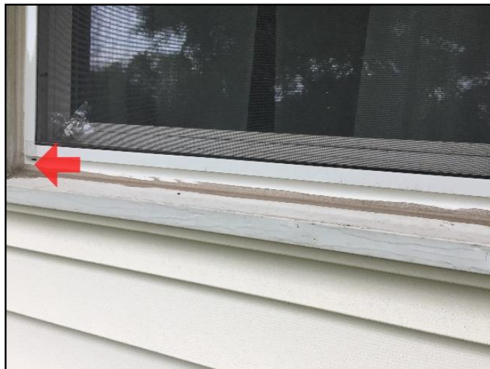
Paint and Caulking - deteriorated / missing
