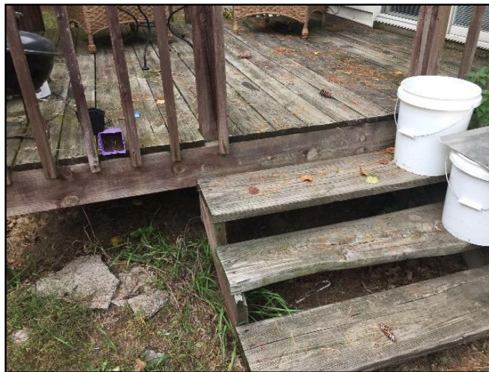
Missing hand rail on deck
