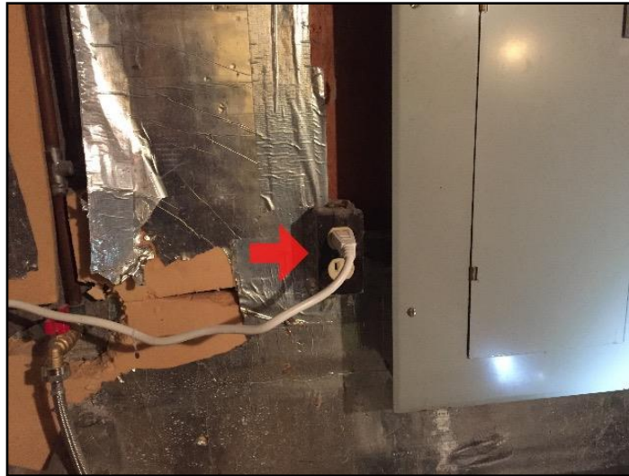
GFCI/GFI needed (Ground Fault Circuit...
