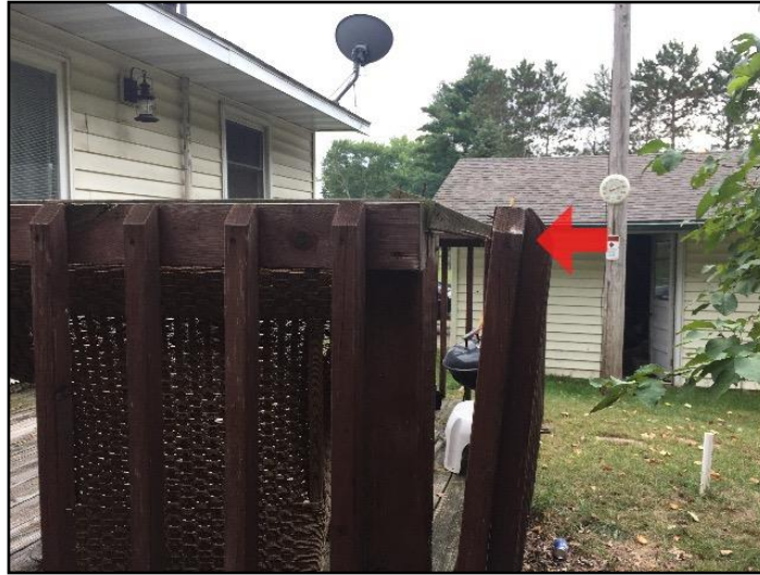
Loose guard rail on deck.
