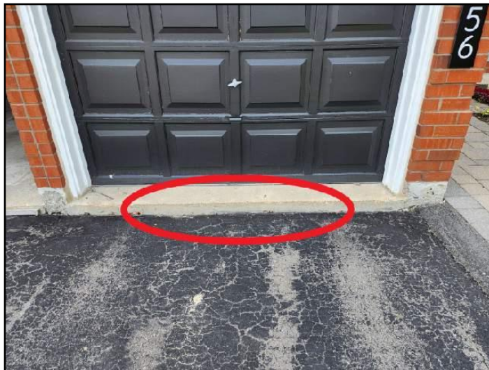
6. Driveway dropped/ settled at garage entry...
