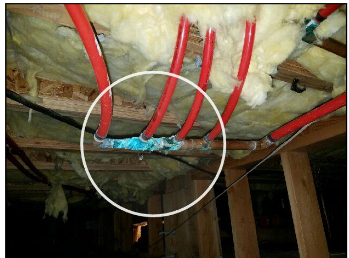
Corrosion/loose
