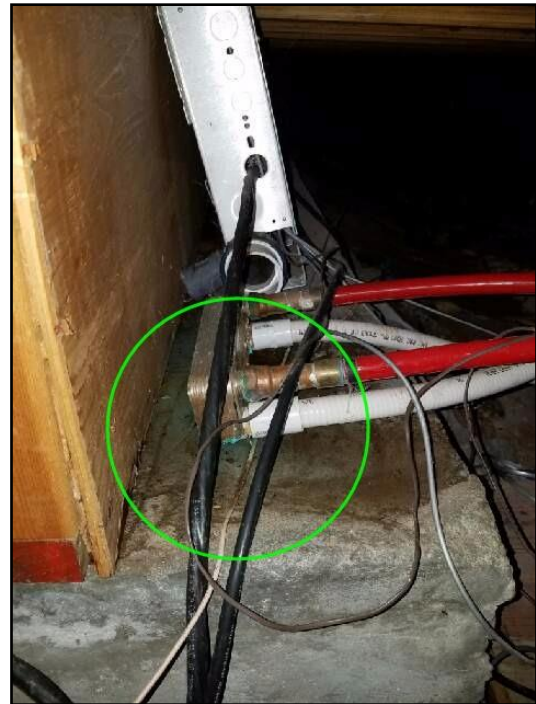
Active leakage
