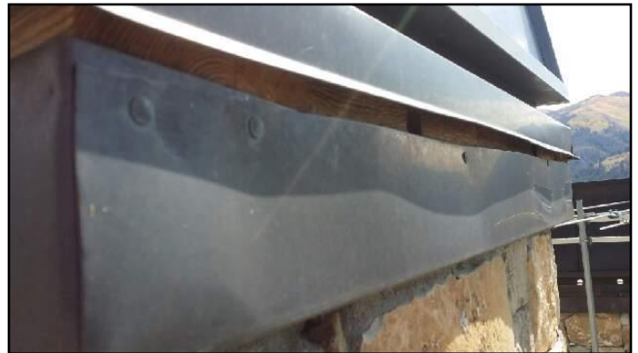
Gap in flashing
