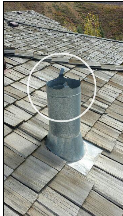
Missing weather cap
