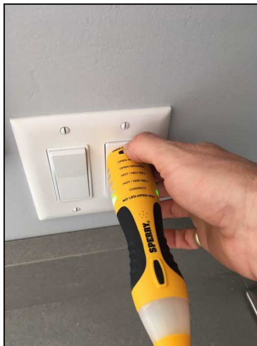
No GFCI/GFI (Ground Fault Circuit...
