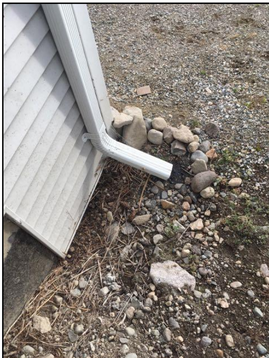
Should discharge 6 feet from building
