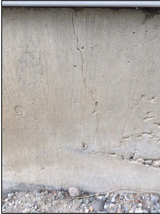
Typical shrinkage crack
