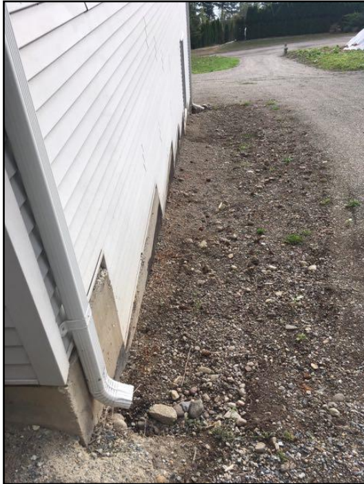
Should discharge 6 feet from building
