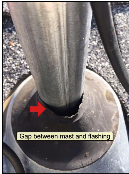
Loose Flashing
