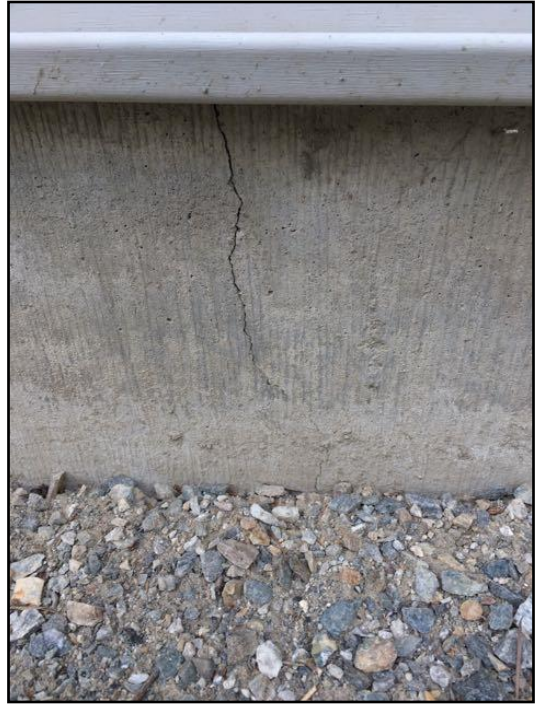
Typical shrinkage crack
