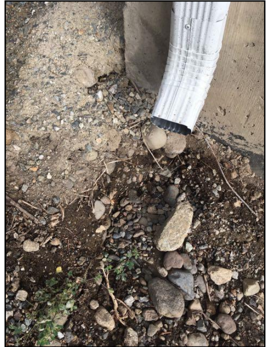
Should discharge 6 feet from building
