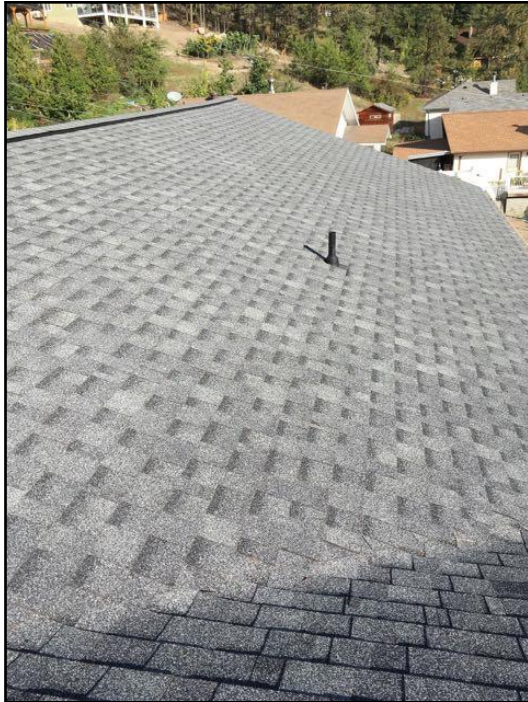
Asphalt shingles
