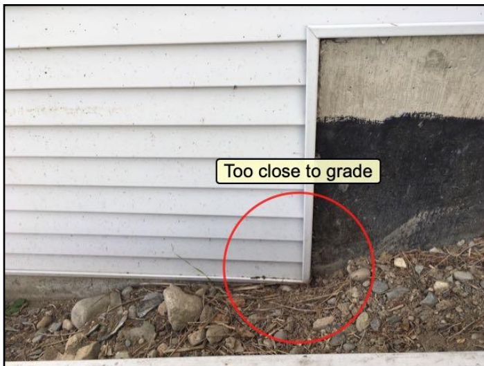
Too close to grade or wood/soil contact
