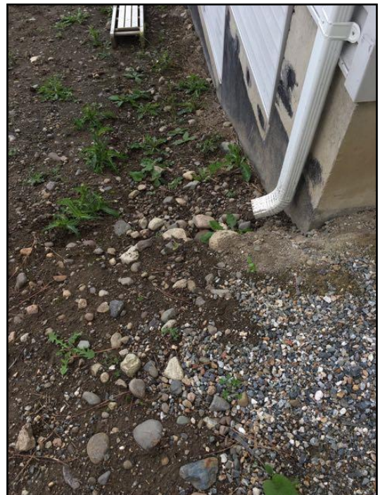
Should discharge 6 feet from building
