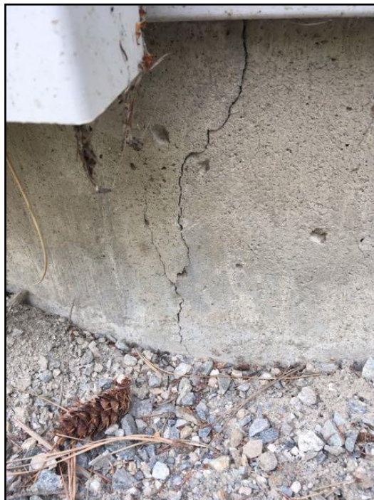
Typical shrinkage crack
