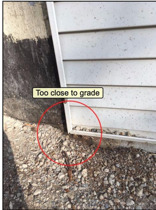
Too close to grade or wood/soil contact
