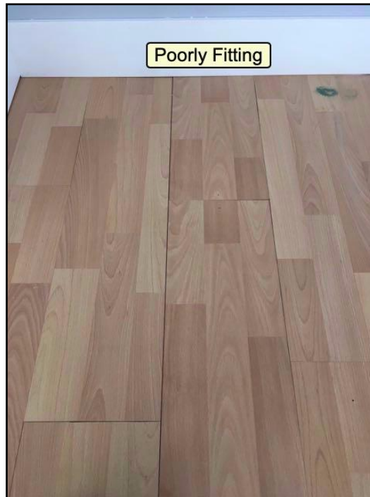
Laminate flooring not tight
