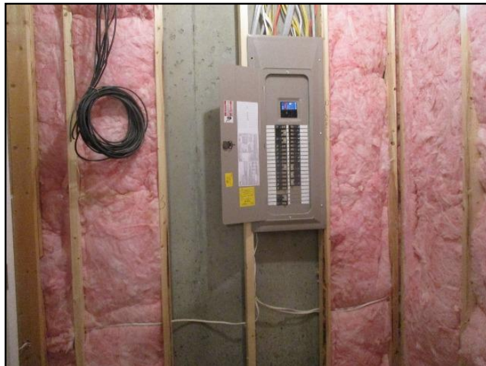
32. Missing Insulation
