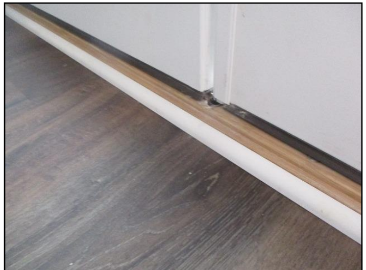
8. Doors not aligned and with gap
