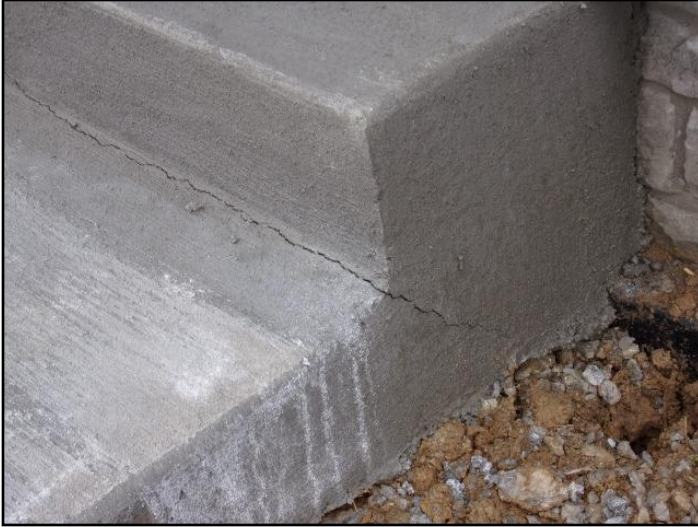
14. Cracked front steps
