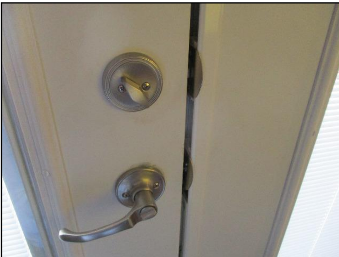
7. Damaged door latch
