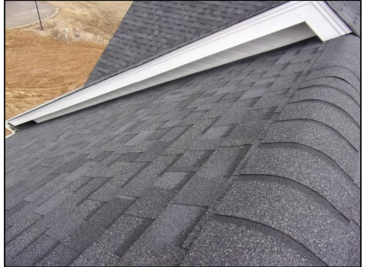
2. Asphalt shingles
