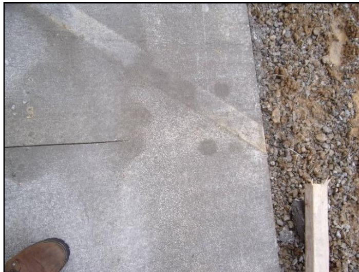
16. Saw joint incomplete
