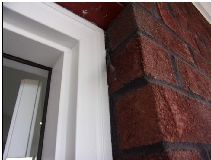
10. Caulking missing, deteriorated or loose
