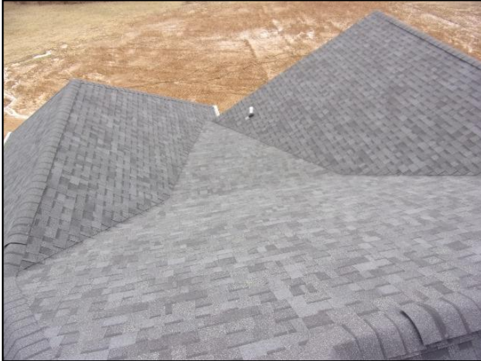
1. Asphalt shingles
