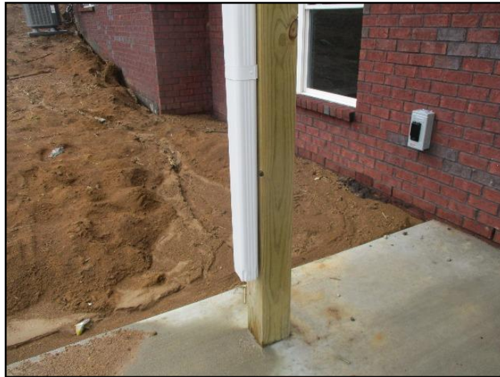
6. Missing elbow and discharge
