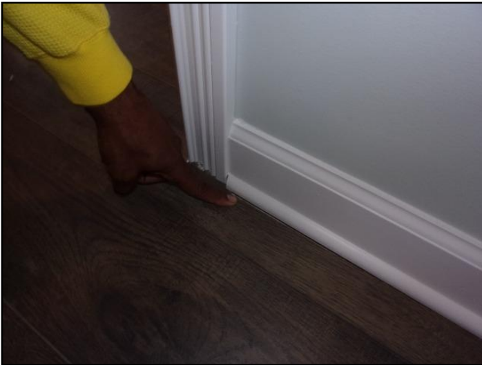
46. Improper installation
