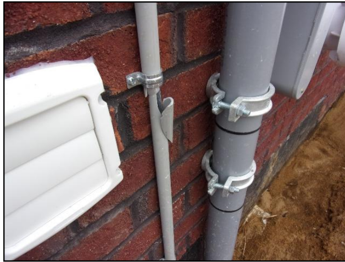
20. Damaged grounding conduit
