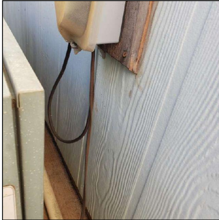
Extension cord used as permanent wiring
