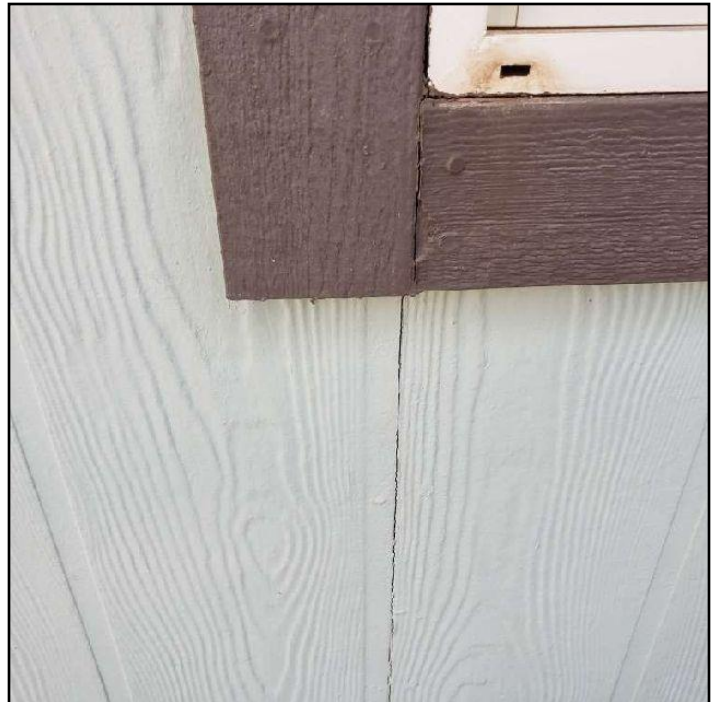
Missing paint or caulking
