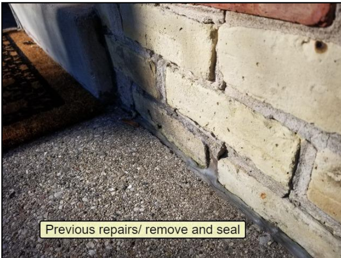
42. Improper slope or drainage
