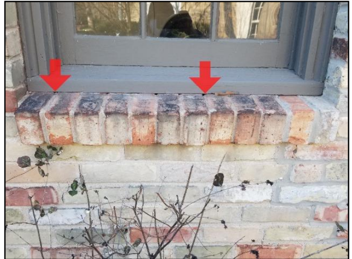
37. Caulking loose, missing or deteriorated
