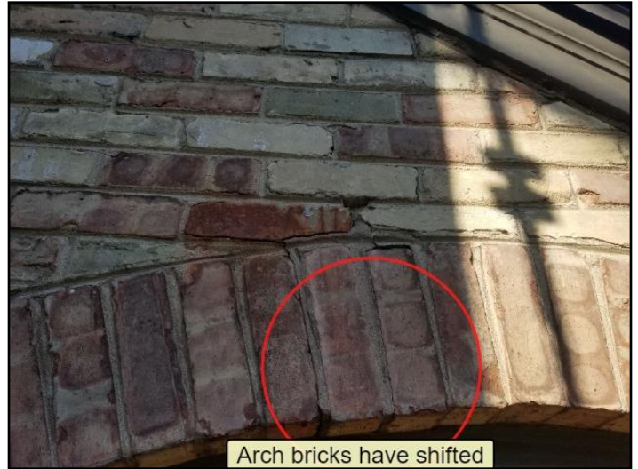
27. Masonry deterioration
