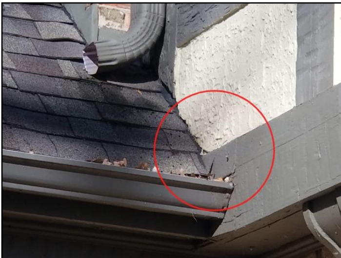
11. Kickout flashing - missing
