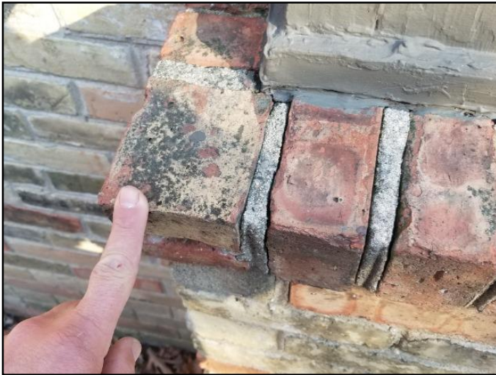
28. Masonry deterioration
