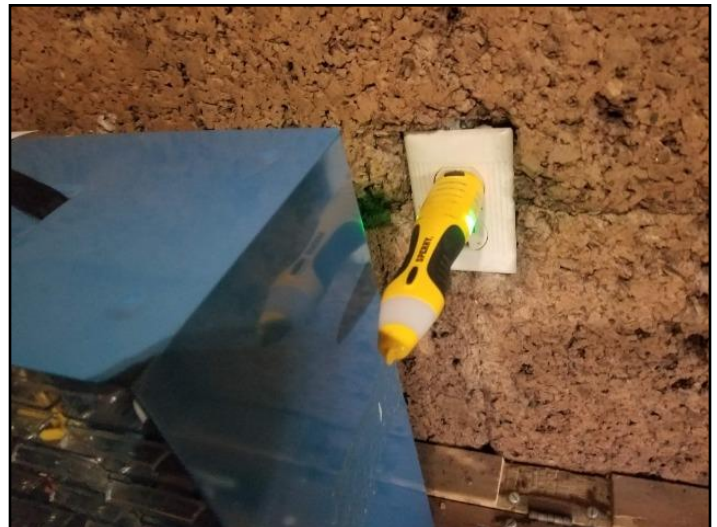
63. GFCI/GFI needed (Ground Fault Circuit...
