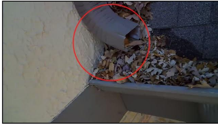
13. Kickout flashing - missing
