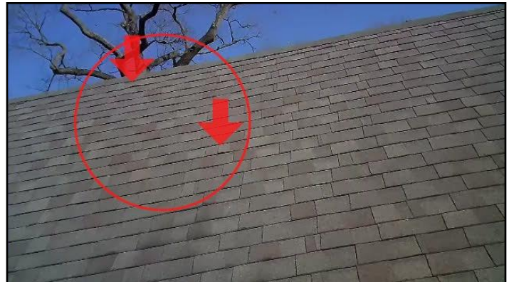
6. Nail Pop Have roofer or handyman correct...
