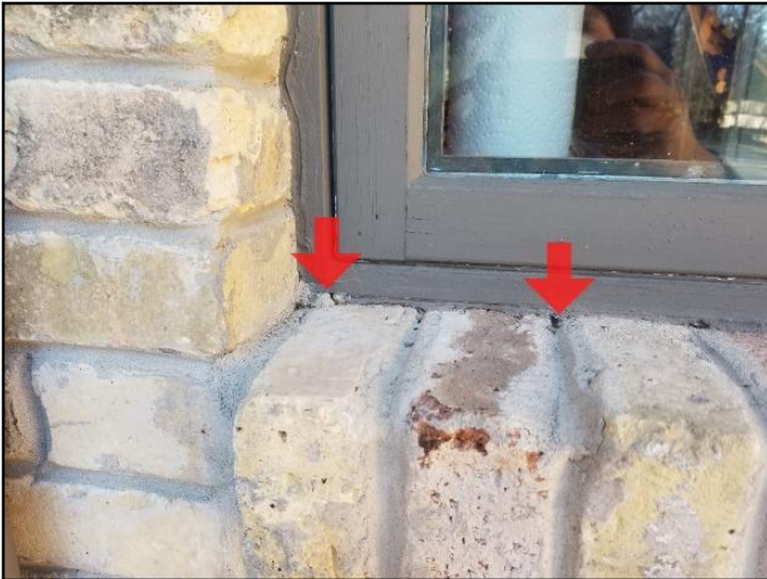
36. Caulking loose, missing or deteriorated
