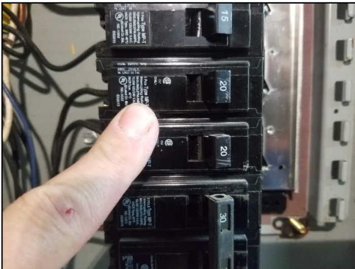
47. Breaker bridge missing
