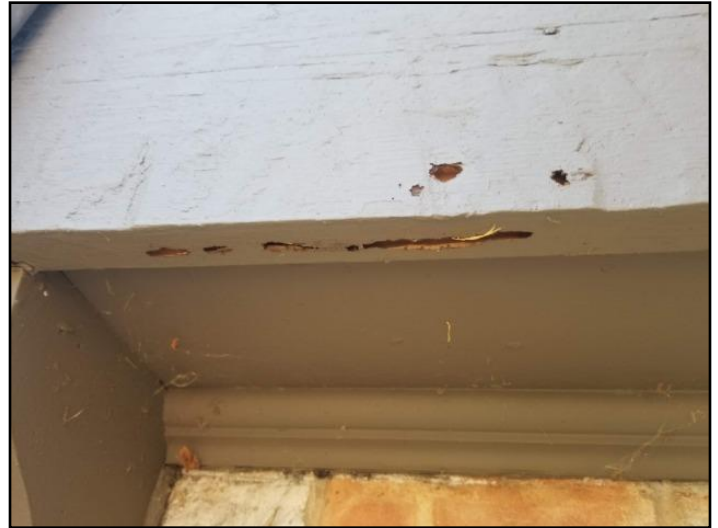
21. Rot or insect damage
