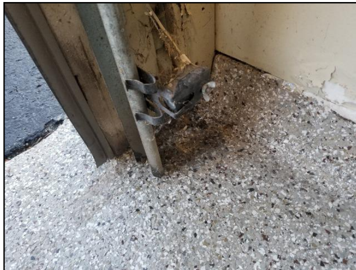
82. Sensors poorly located
