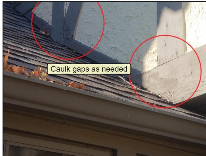
22. Caulking missing or deteriorated
