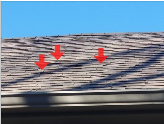
5. Nail Pop Have roofer or handyman correct...
