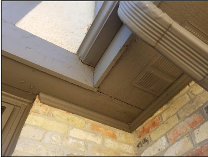
20. Rot or insect damage
