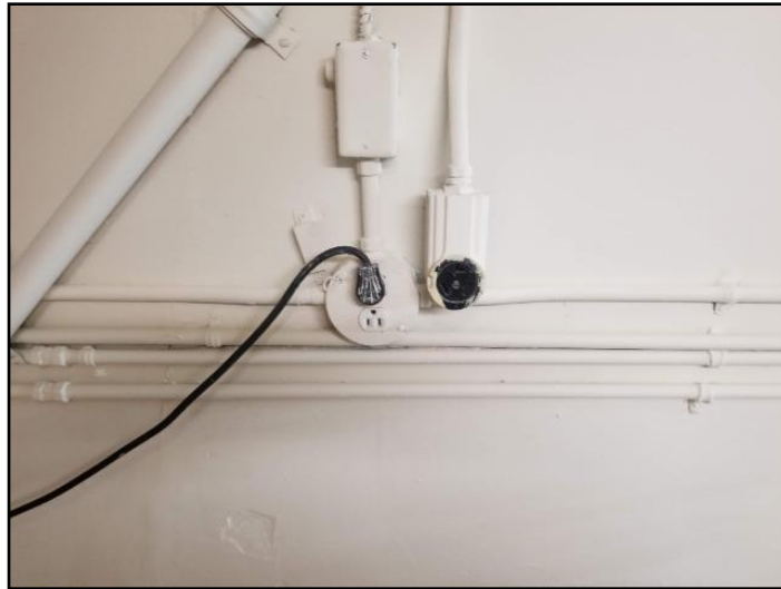
64. GFCI/GFI needed (Ground Fault Circuit...
