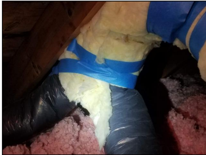
80. Multiple ducts are combined to a single...
