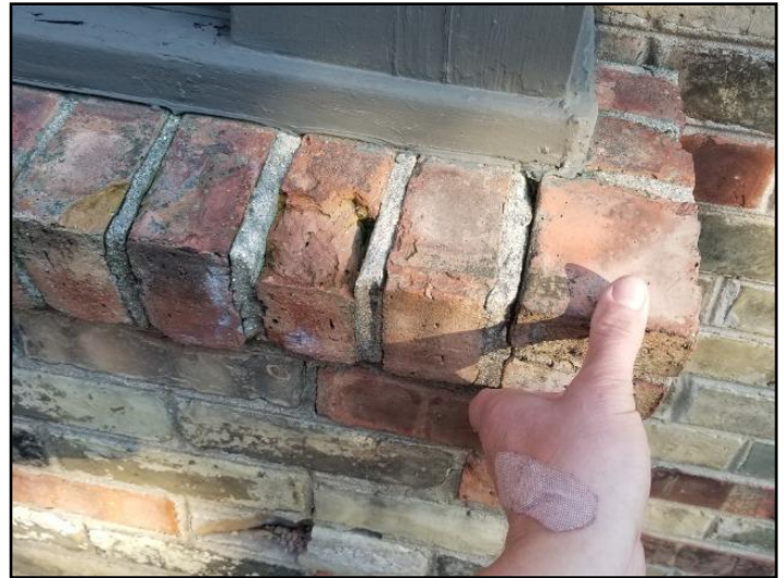
29. Masonry deterioration
