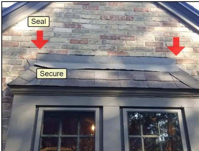
7. Damage, loose, open seams, patched
