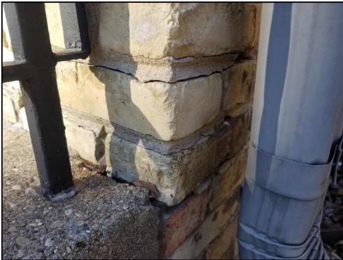
32. Mortar deterioration
