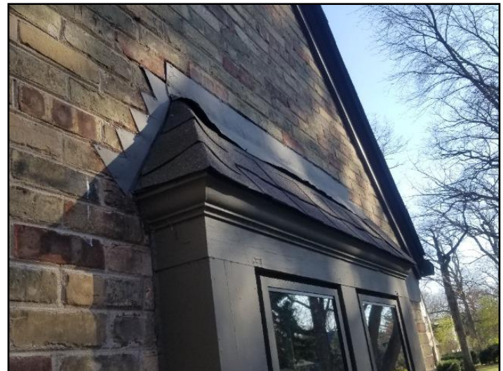
8. Damage, loose, open seams, patched
