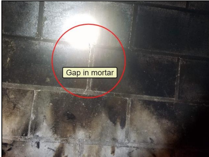
70. Deteriorated, missing or loose masonry or...
