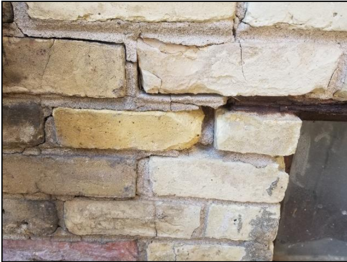
26. Masonry deterioration
