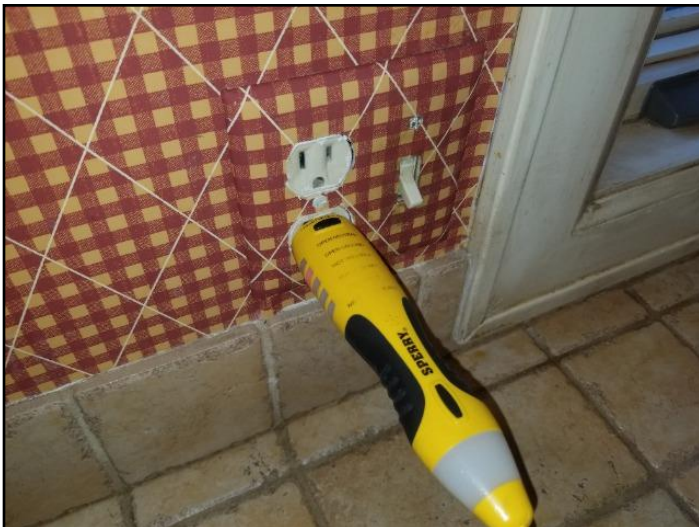
62. GFCI/GFI needed (Ground Fault Circuit...
