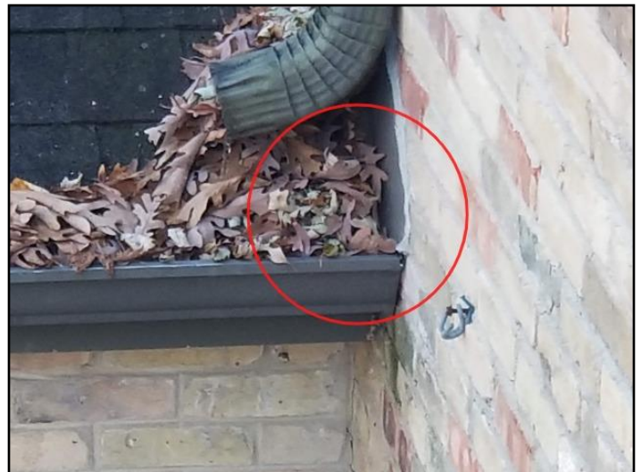
12. Kickout flashing - missing
