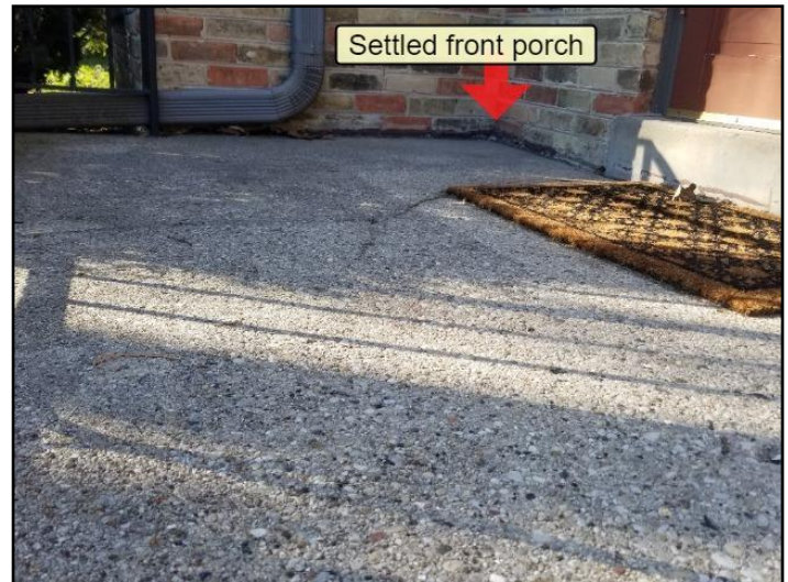
43. Improper slope or drainage
