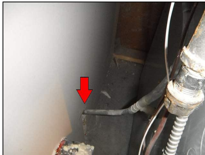
Condensate Line - poorly routed to drain
