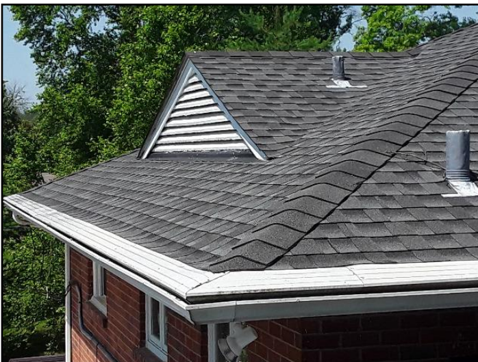
3. Asphalt shingles
