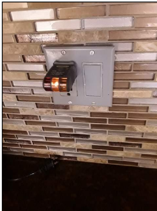
21. Test faulty on GFCI
