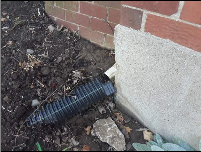
9. Loose connections
