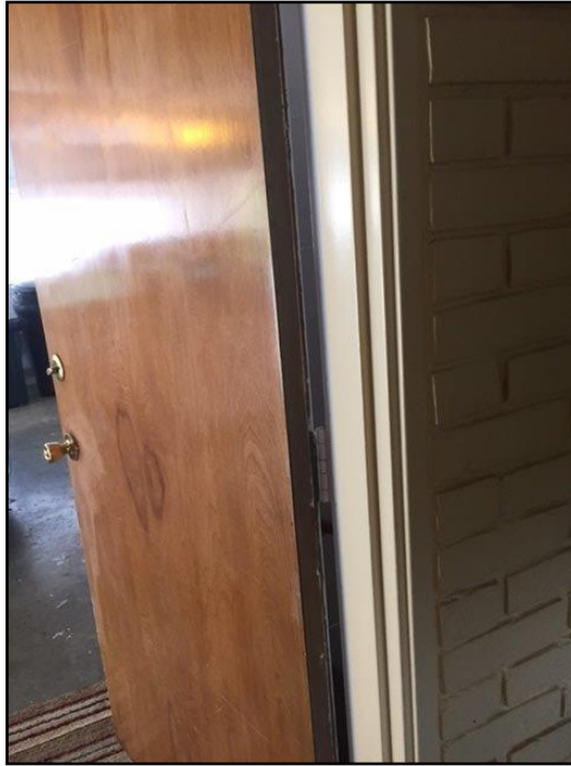
17. Garage door not fire rated
