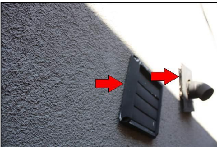
7. Caulking missing or ineffective
