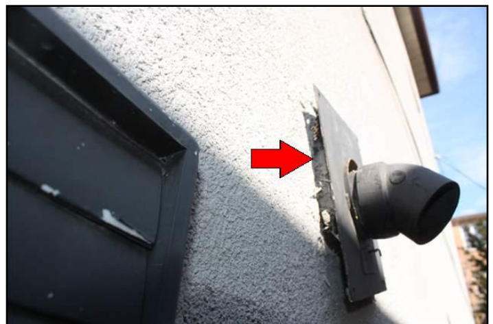
8. Caulking missing or ineffective
