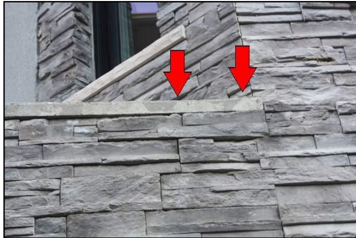
6. Flashings missing
