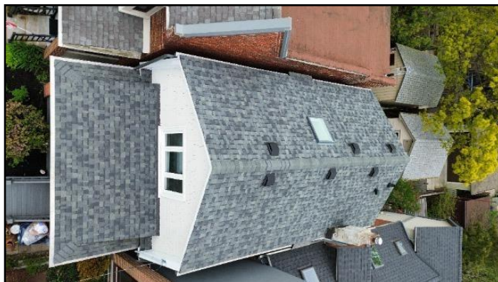
2. Asphalt shingles -- Good condition
