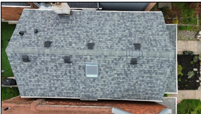
1. Asphalt shingles -- Good condition
