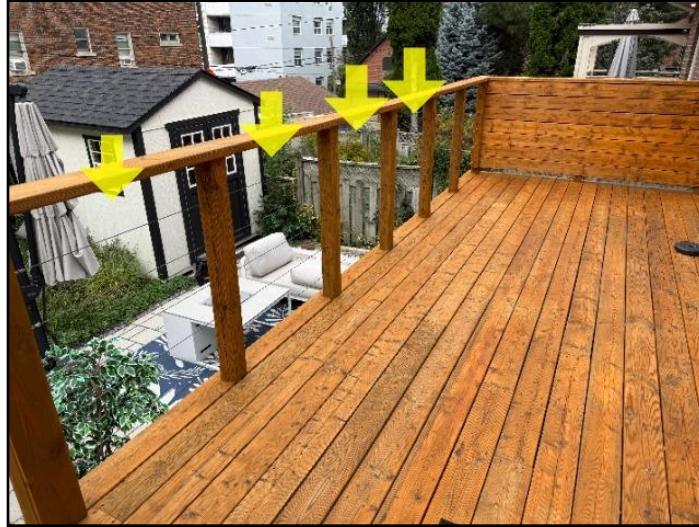
9. Horizontal cable guard infill flexible /...
