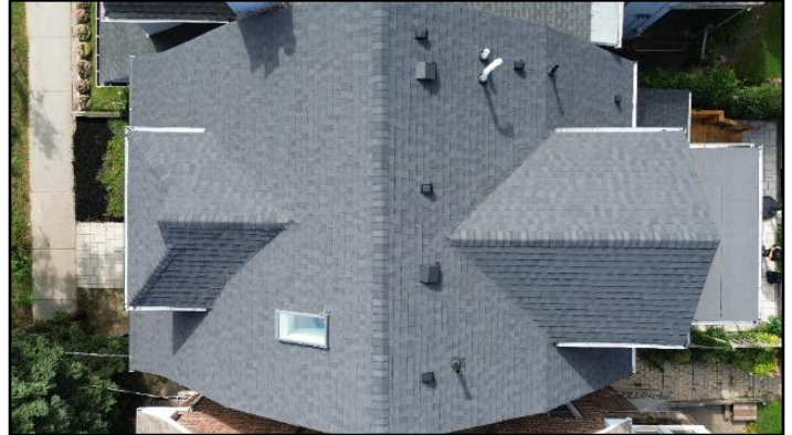
2. Asphalt shingles -- Good condition
