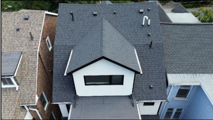
1. Asphalt shingles -- Good condition
