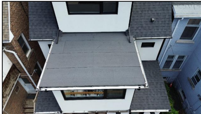
3. Modified bitumen membrane
