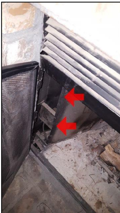
Flashing missing
