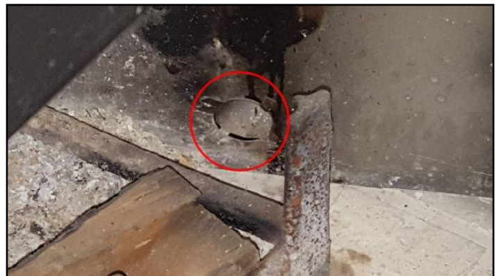
Gas line opening not sealed shut
