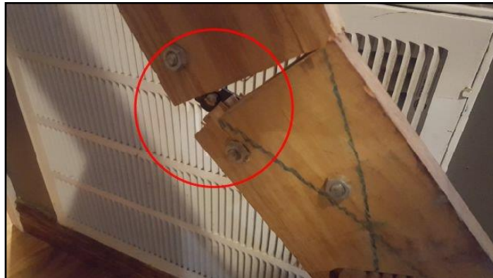
Treads loose or broken
