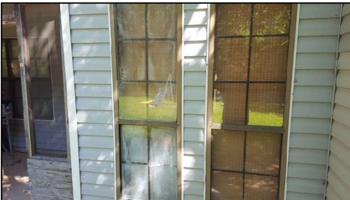
Lost seal on double glazing
