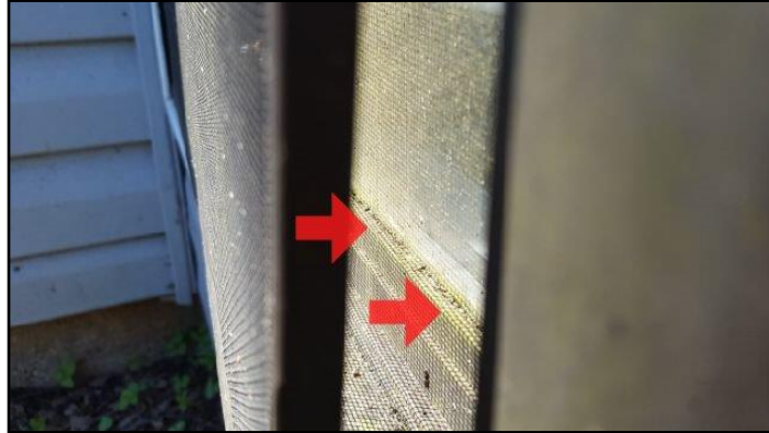
Caulking loose, missing or deteriorated
