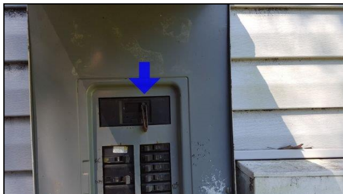
Main electrical shut off
