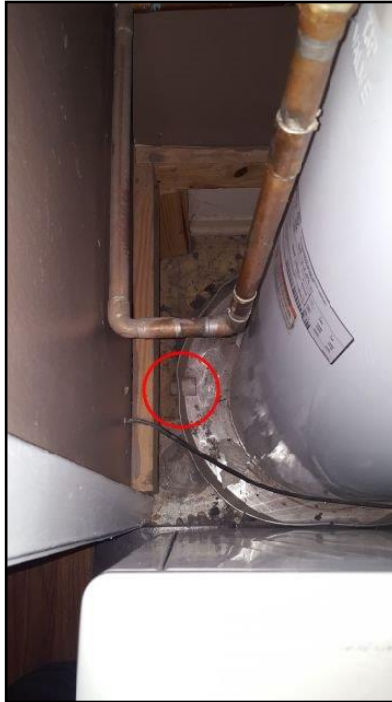
Missing catch pipe
