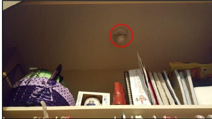
Improper closet lighting
