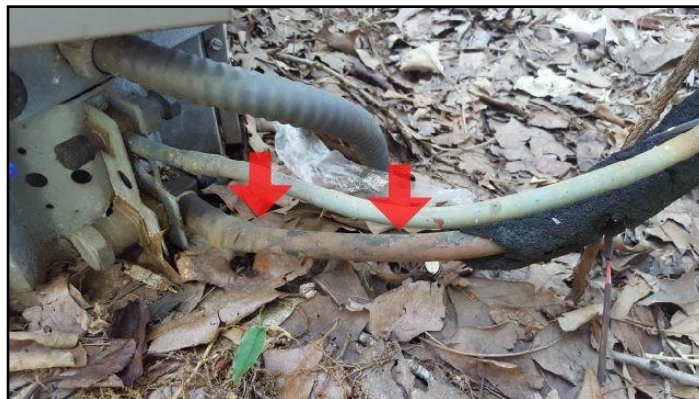
Insulation - missing
