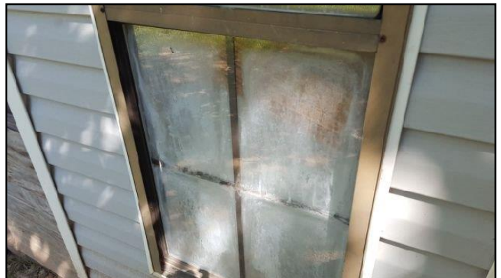
Lost seal on double glazing
