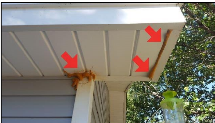
Excess use of spray foam
