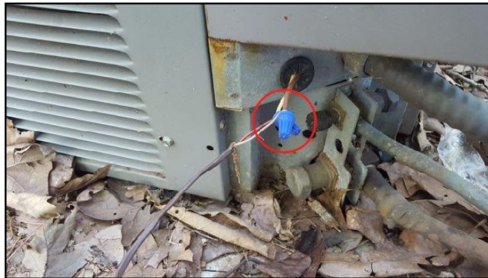
Exposed electrical wires and splices
