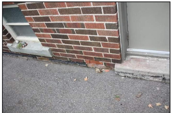
6. Spalling
