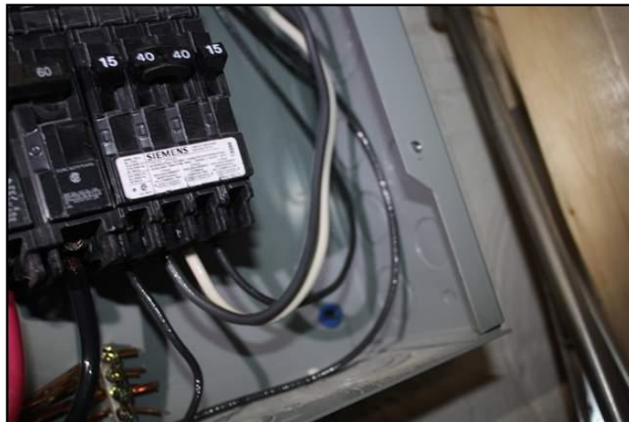
25. Improper color coding
