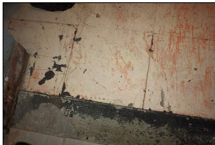
42. Possible asbestos containing materials
