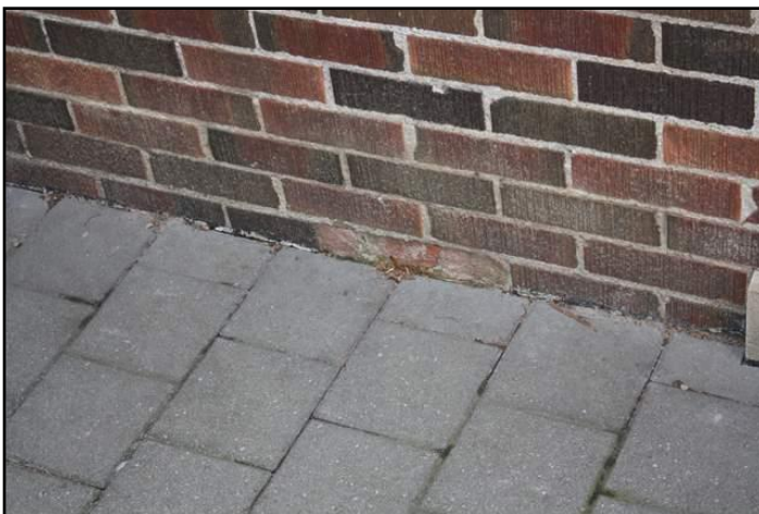
5. Spalling
