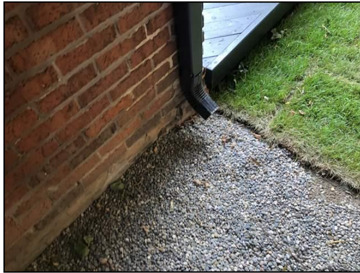
3. Should discharge 6 feet from building
