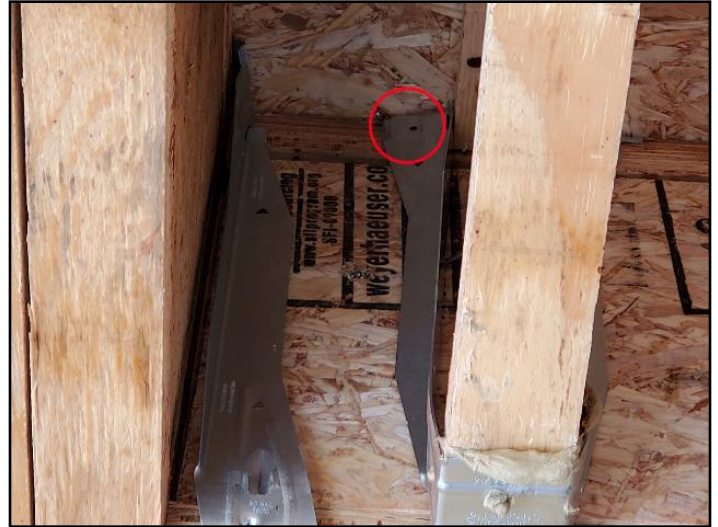
Poor end bearing, joist hanger connections
