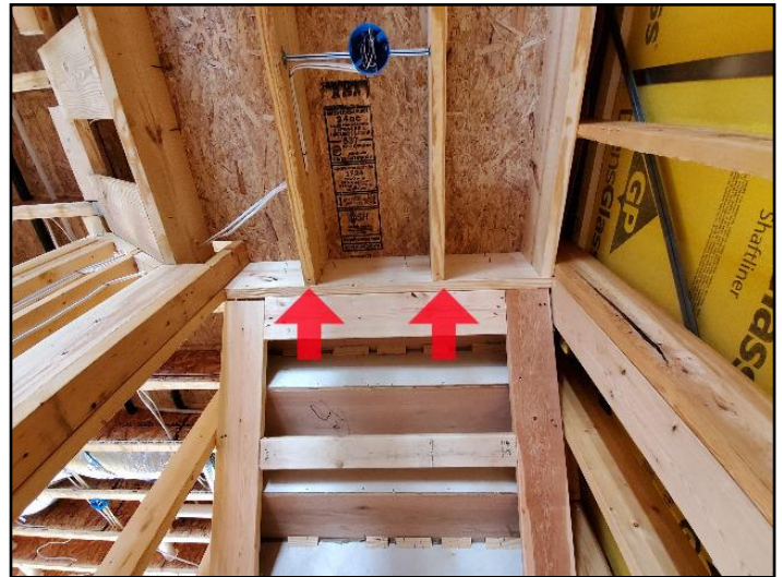
Poor end bearing, joist hanger connections
