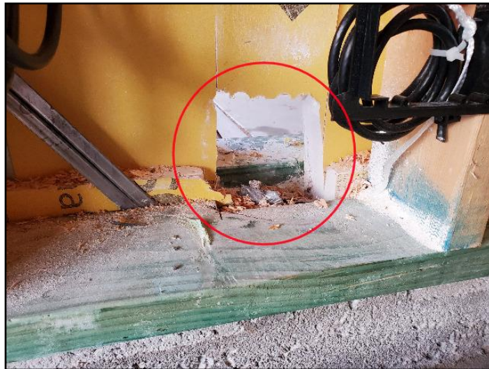
Hole in firewall
