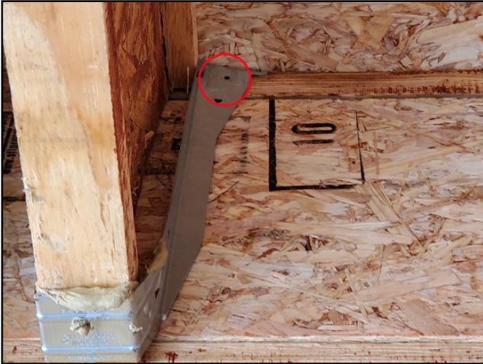
Poor end bearing, joist hanger connections
