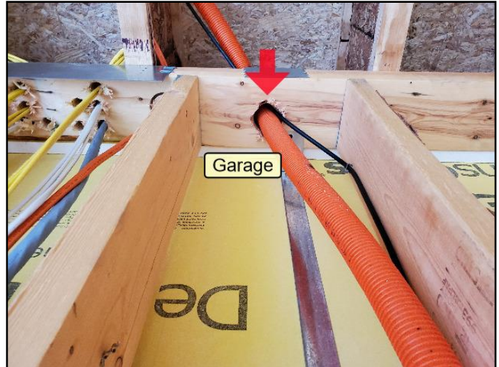
penetrations in top and bottom plates
