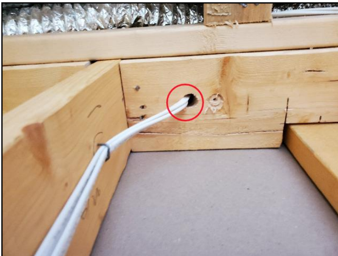
Penetrations in top and bottom plates
