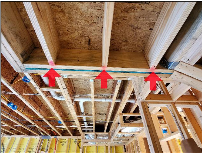
Poor end bearing, joist hanger connections
