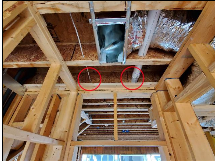
Fire separation between garage and living...
