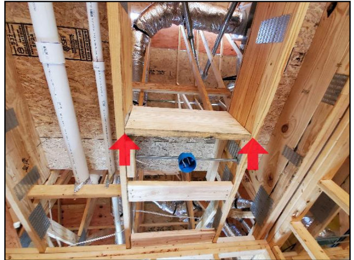
Poor end bearing, joist hanger connections
