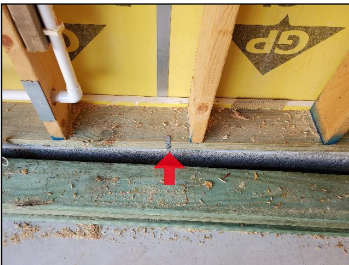
Anchor bolts missing
