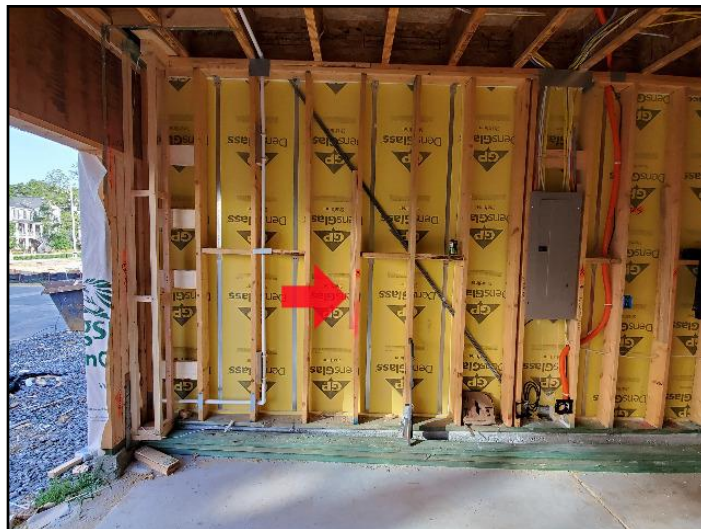
Leaning, bowing, buckling
