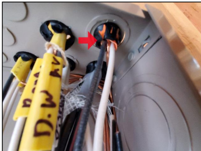
Sheath into the panel
