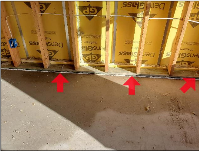
Anchor bolts missing
