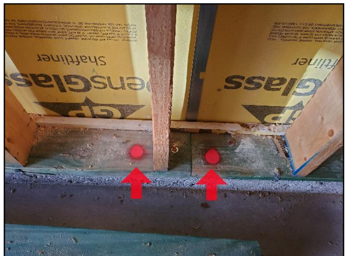
Anchor bolts missing
