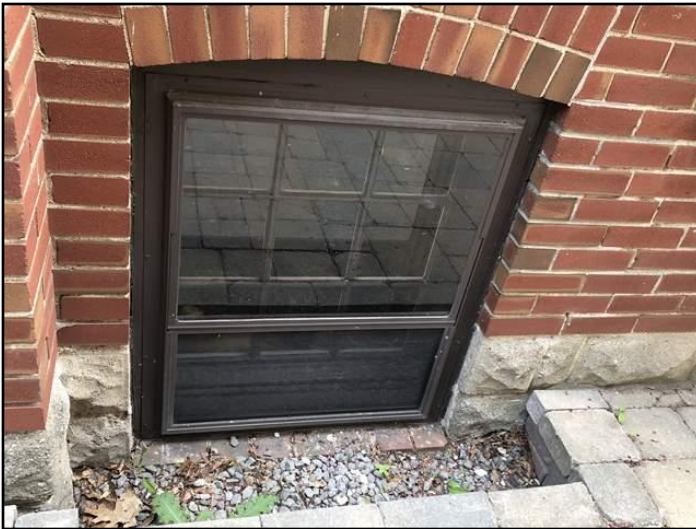
11. Less than 6 inches below window
