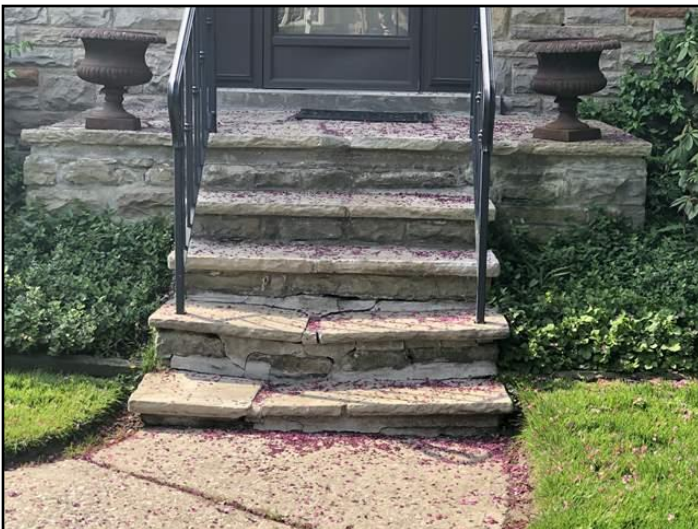
17. Steps or landings settling or heaving
