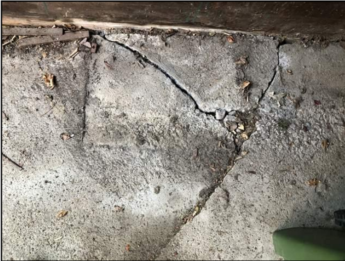
19. Cracked and settled
