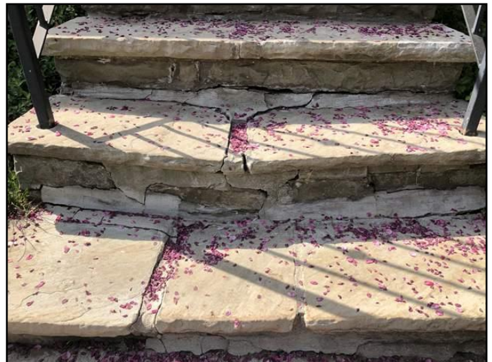
18. Steps or landings settling or heaving
