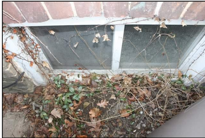
17. Sill - Near or at Grade Level
