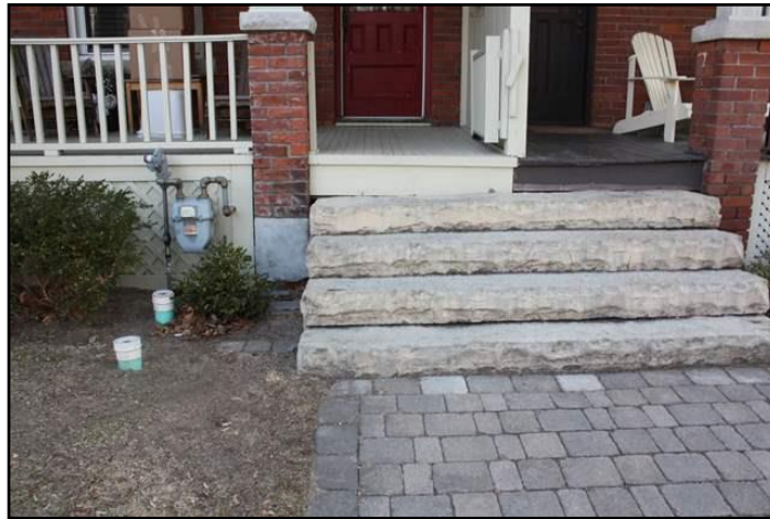
19. Steps or landings settling or heaving
