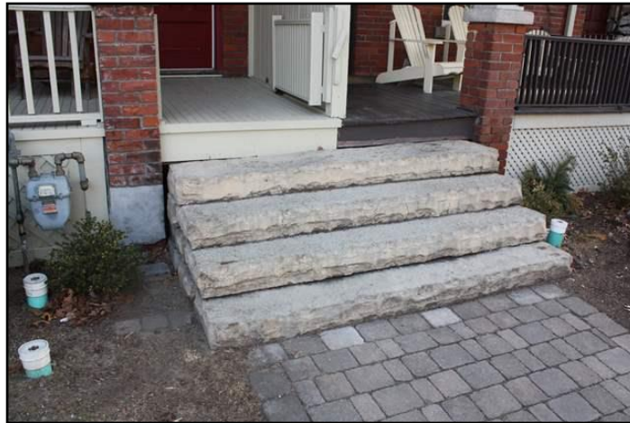
20. Missing Handrail
