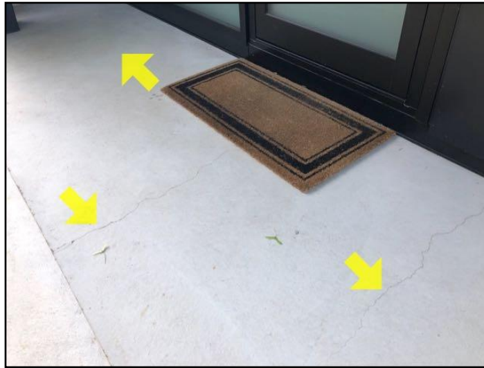
Concrete cracked
