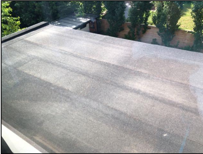
Modified bitumen membrane
