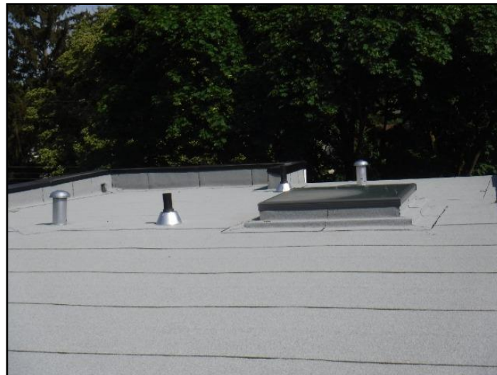
Skylight(s) - vulnerable area for leaks.
