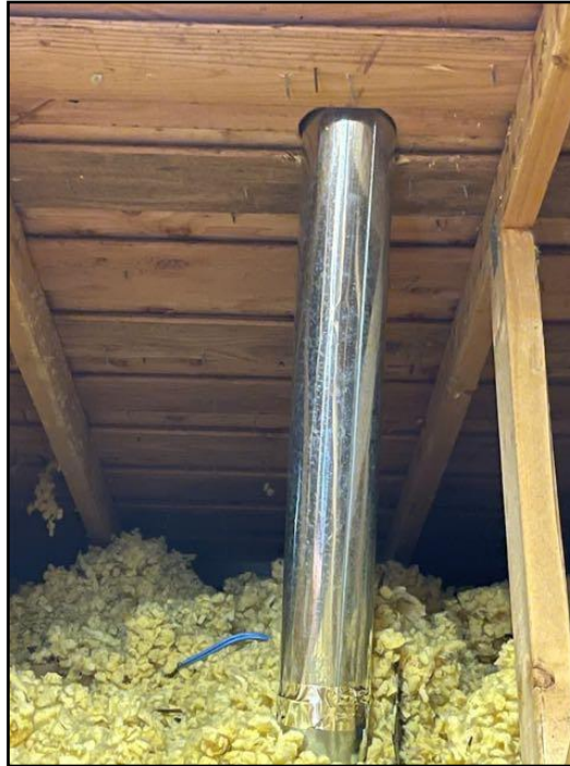
Not insulated in unconditioned space
