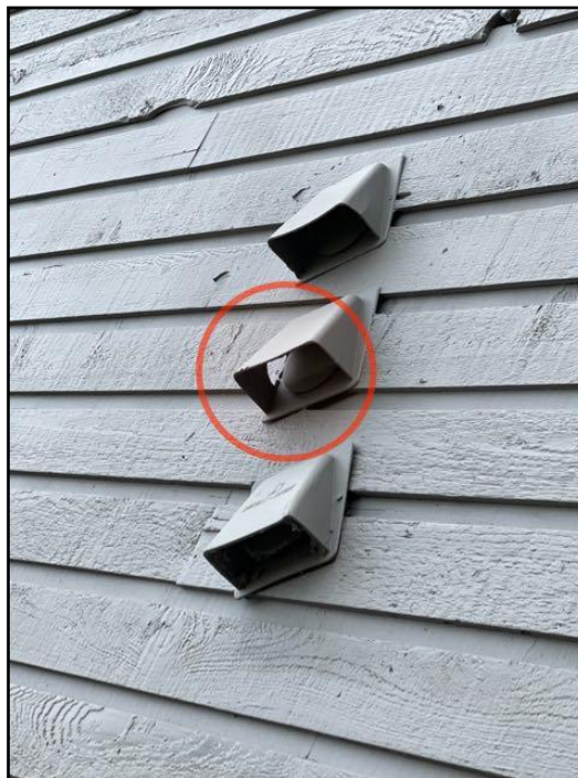
Cover damaged
