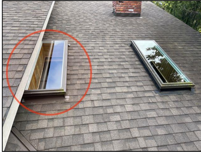
Skylight not well secured
