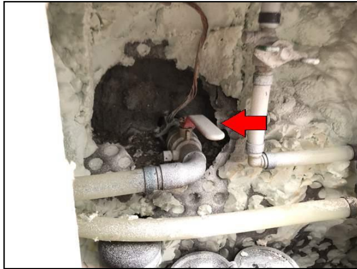
20. Front of the basement
