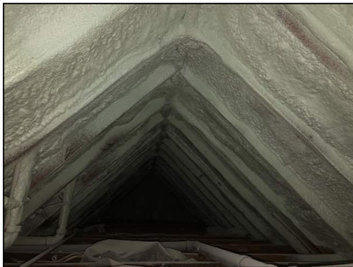
19. Spray foamed attic
