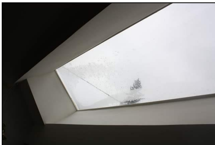
Lost seal on double or triple glazing
