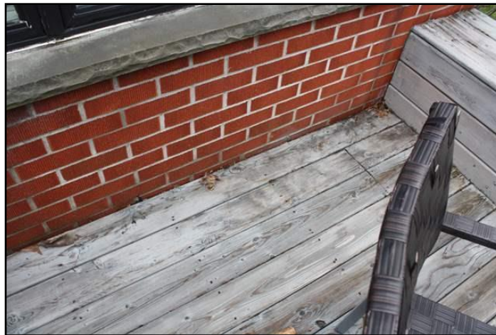
Weep holes missing or ineffective
