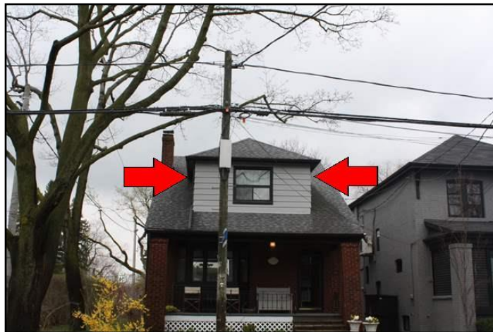
Discharging onto roof
