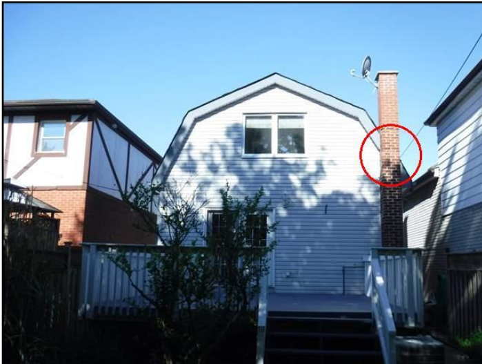
Loose, missing or deteriorated masonry
