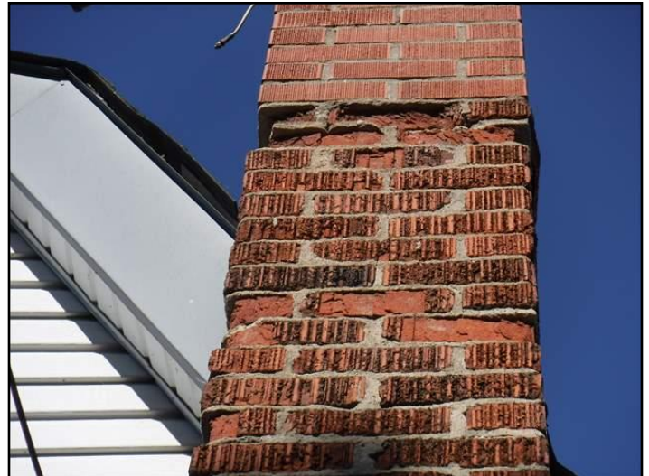
Loose, missing or deteriorated masonry
