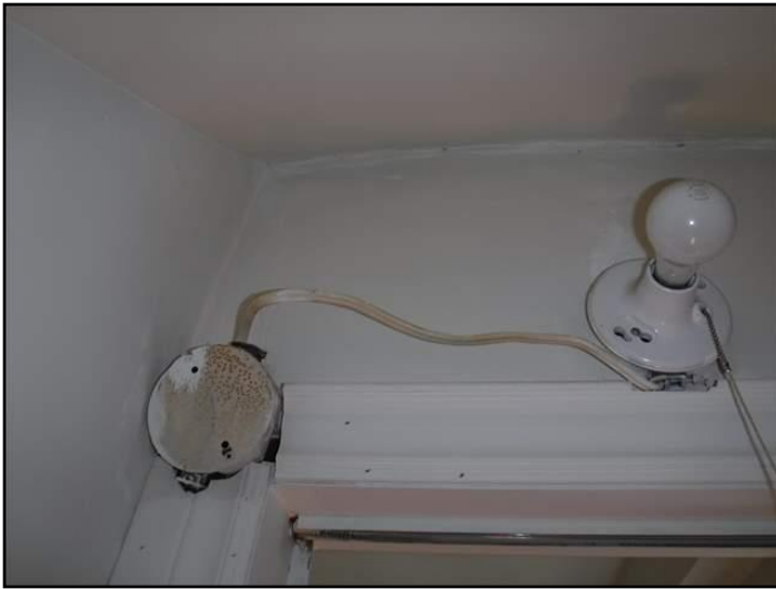
Non-professional installation - exposed wires
