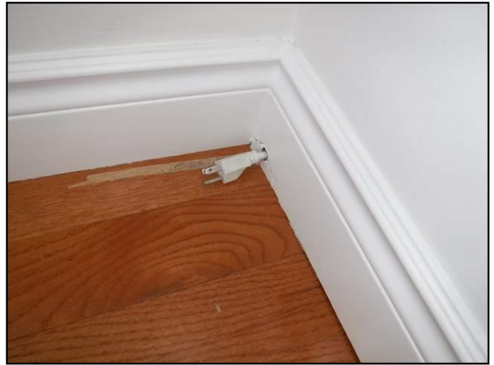
Non-professional installation - through wall
