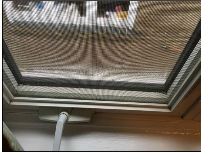
Seal lost on double or triple glazing
