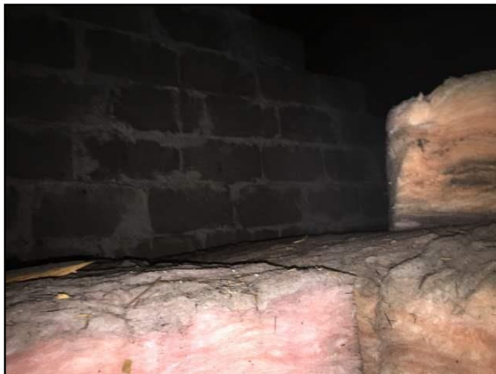
Insulation level below modern standards
