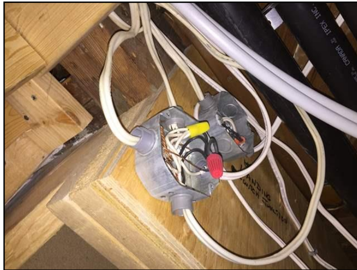
Cover Plate(s) - missing
