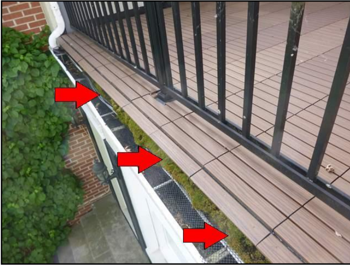
Mossy build-up at edge of flat roof
