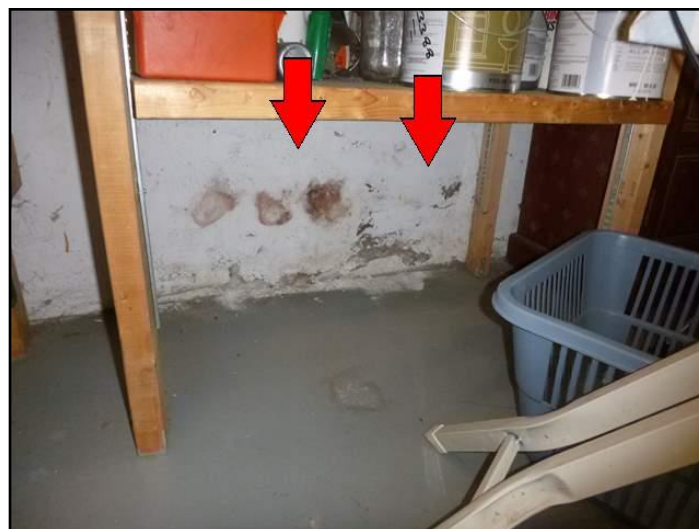
Efflorescence
