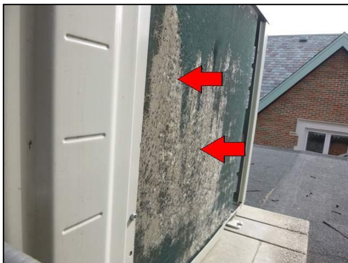
Dirty condenser coil (rooftop unit)
