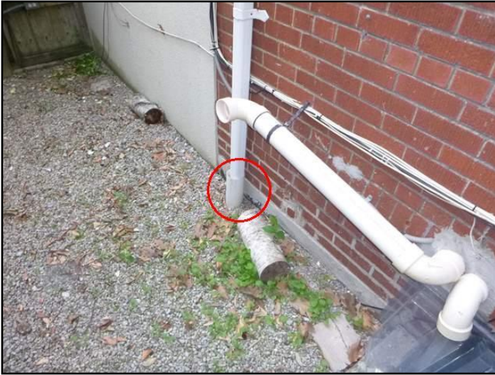
Discharge below grade (rear)
