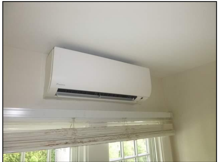
Ductless (Mini split) system- indoor unit
