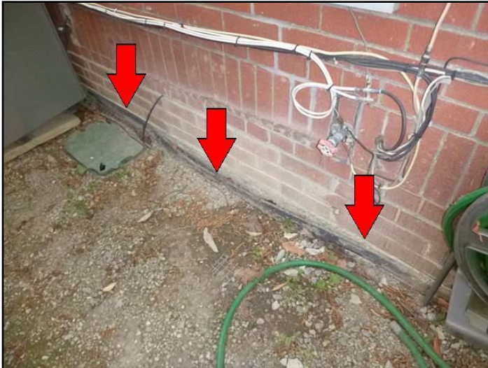
Exterior damp proofing material (west side)
