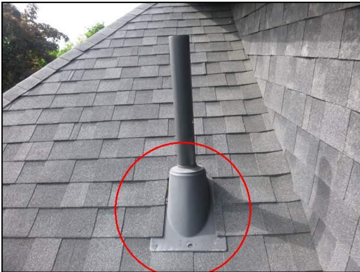
Plumbing stack flashing (circled)
