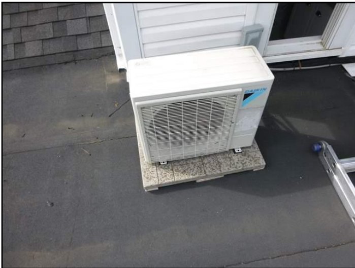
Ductless (Mini split) system- outdoor unit
