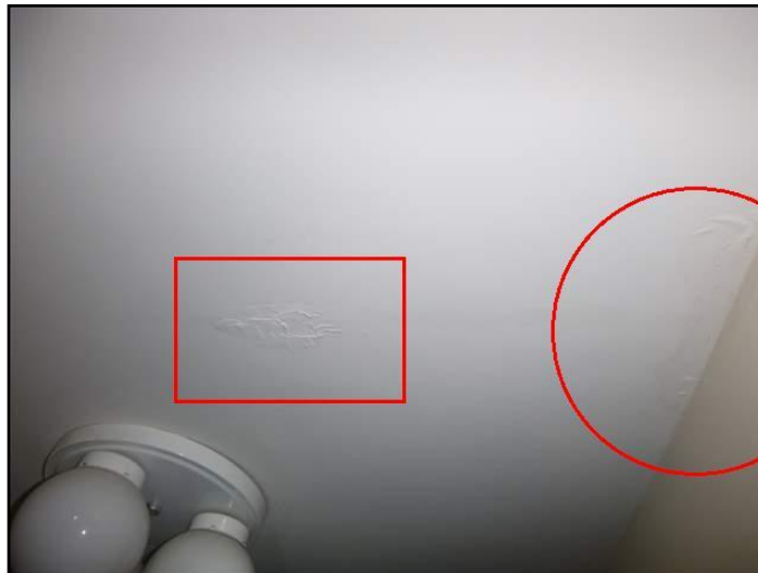
Water damage- dry at inspection
