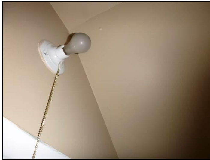
Exposed bulb above closet door
