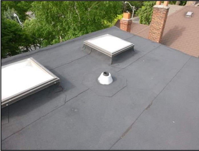
Modified bitumen membrane
