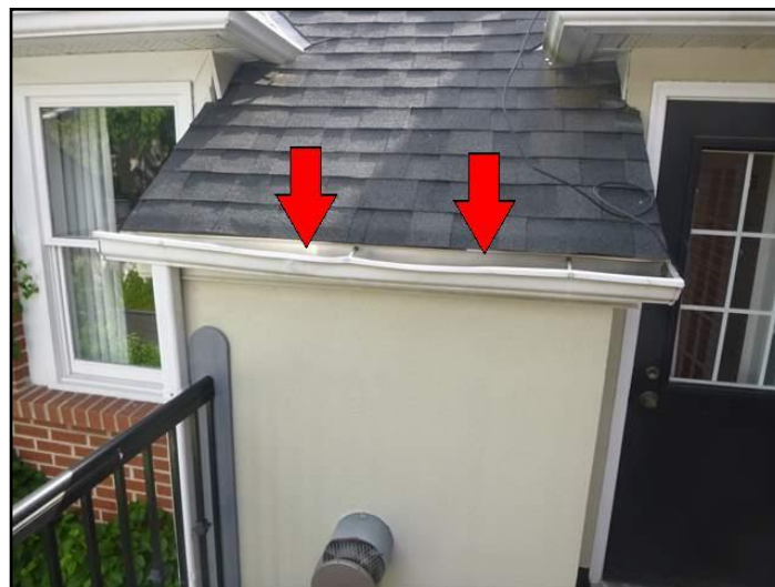
Damaged (bent/sagging) gutter
