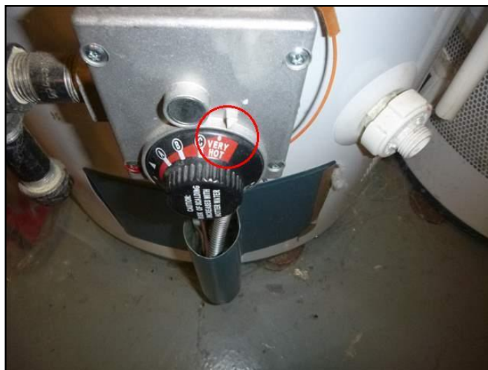
Thermostat set to maximum (typ.)
