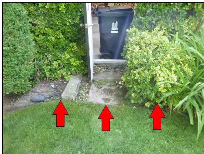
Low area- water drains towards garage
