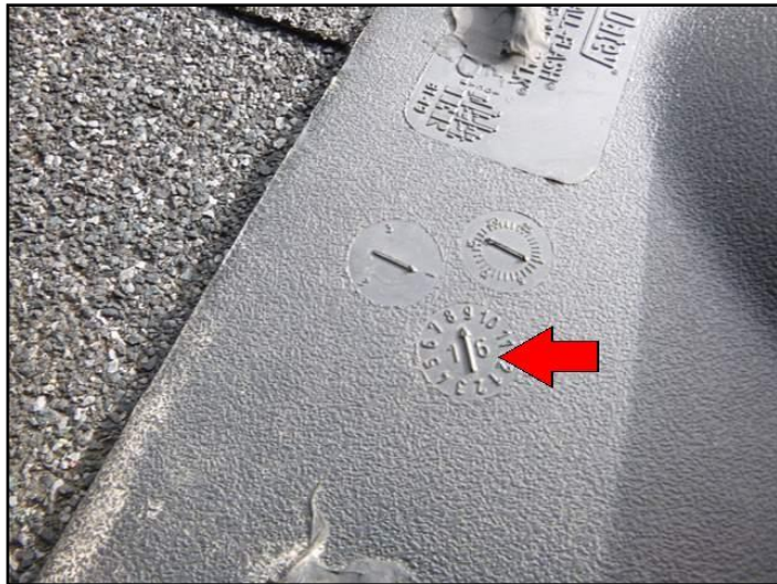
Flashing manufactured in 2016
