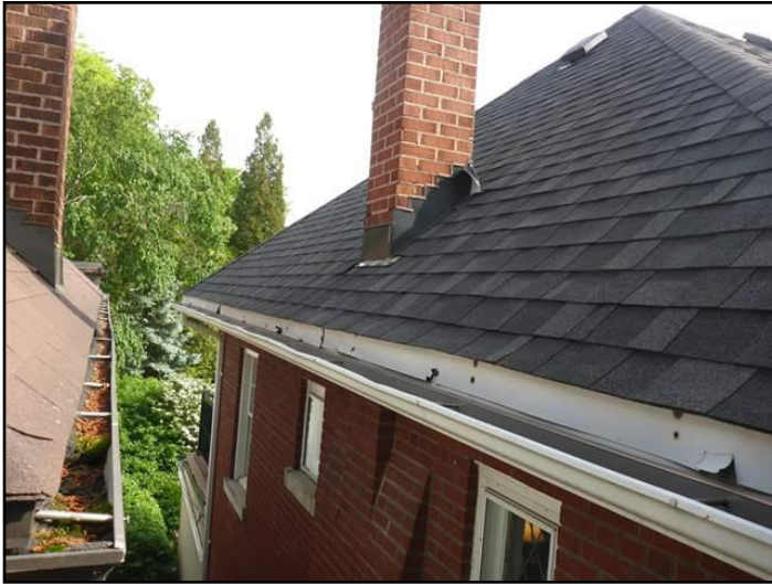
Asphalt shingles
