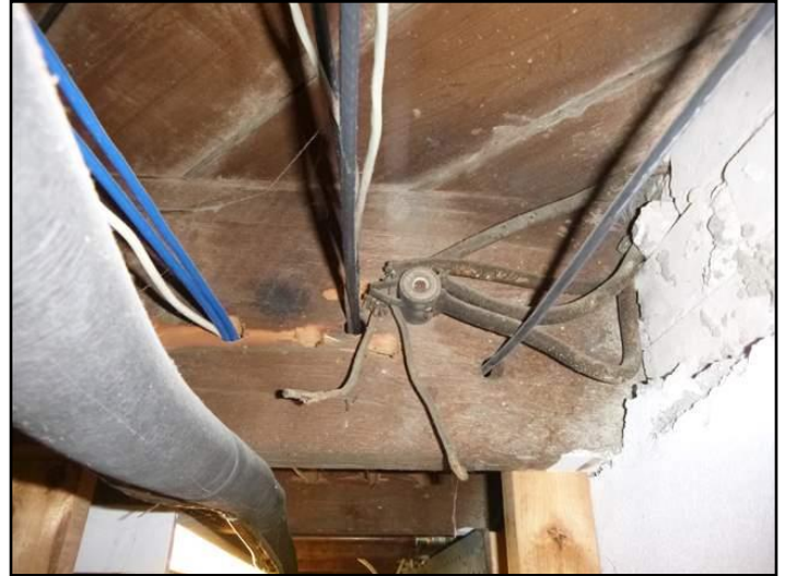
Remnants of knob-and-tube wiring
