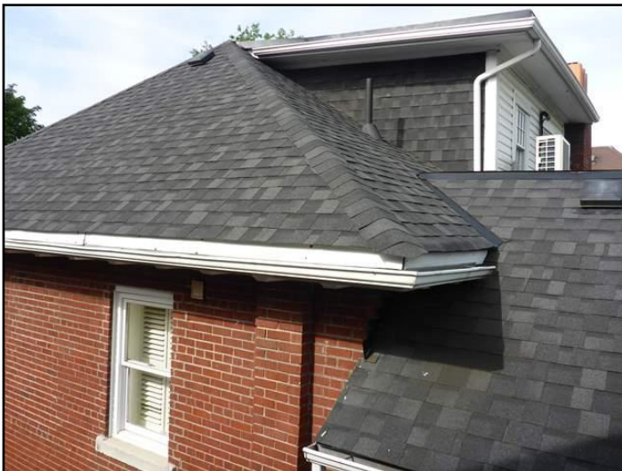
Asphalt shingles
