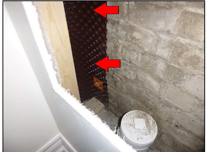
Interior damp proofing membrane (front)
