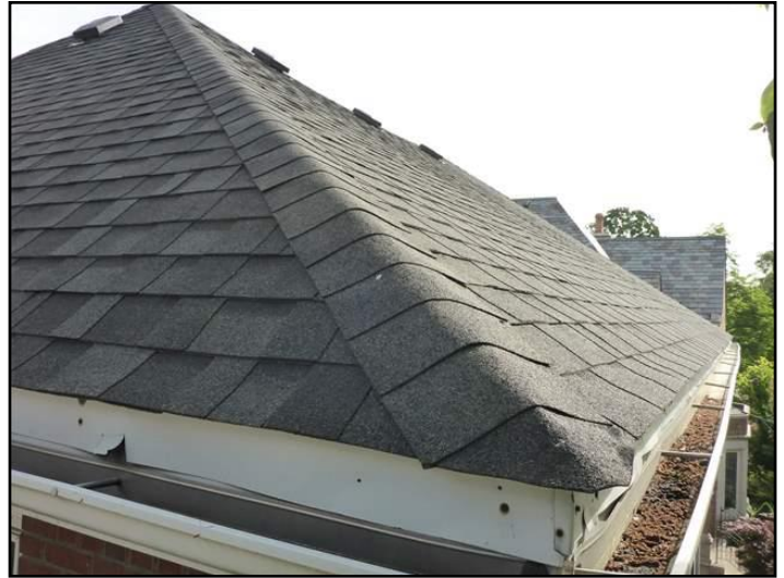
Asphalt shingles
