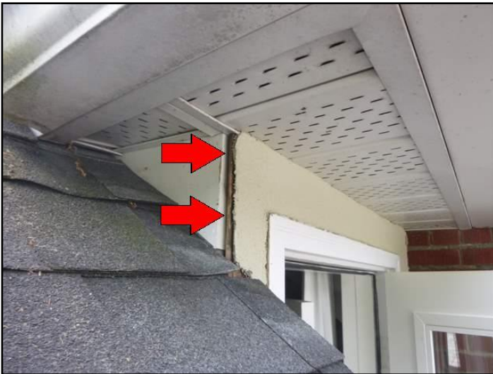
Exposed wood, gaps at second floor walkout
