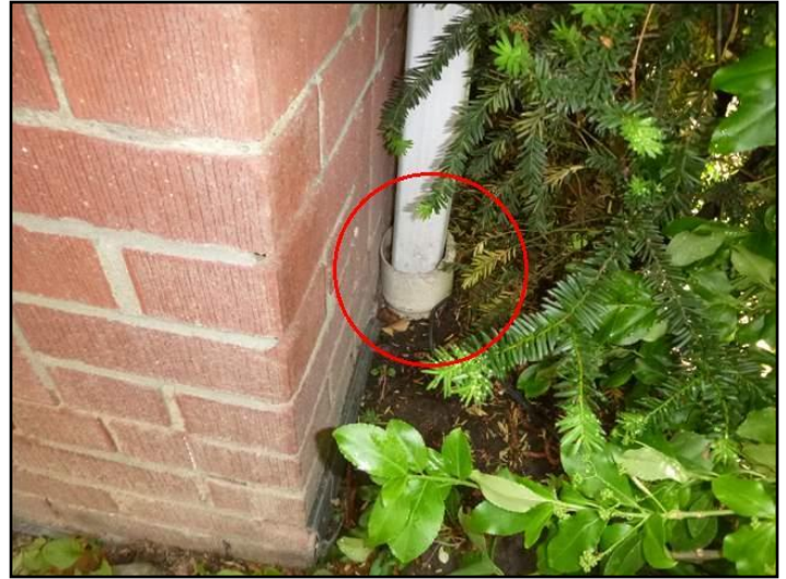
Discharge below grade (front)
