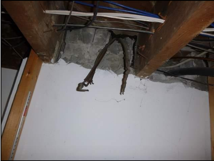
Remnants of knob-and-tube wiring
