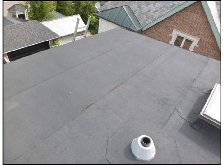
Modified bitumen membrane
