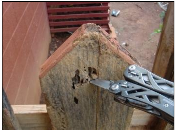
Rot or insect damage
