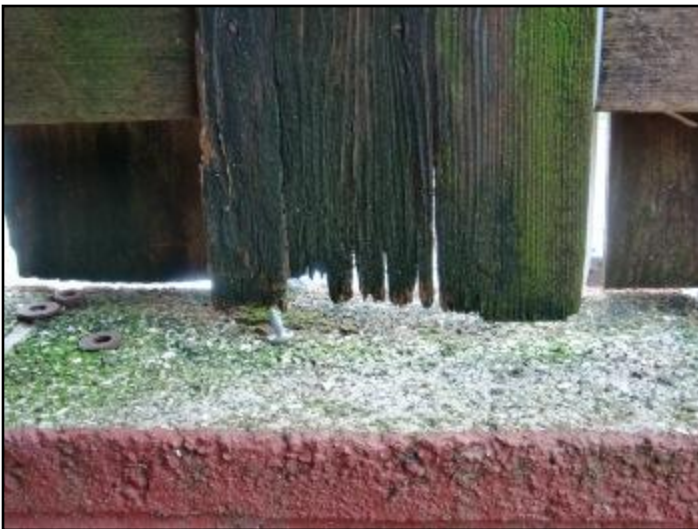
Rot or insect damage
