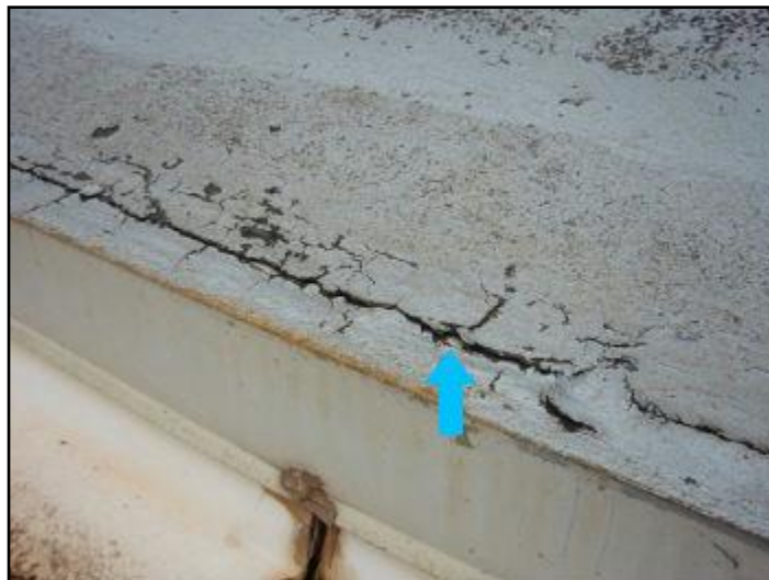
Openings at seams or flashings
