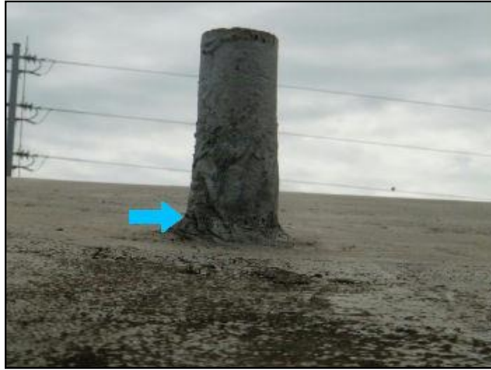
Openings at seams or flashings
