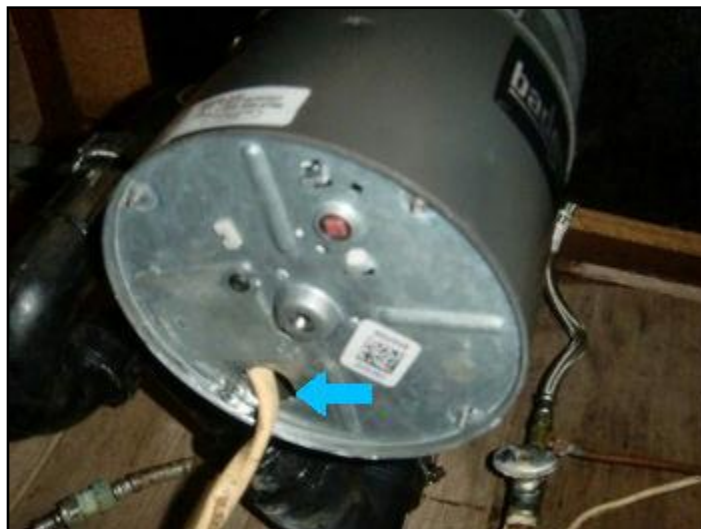
Wiring exposed or loose
