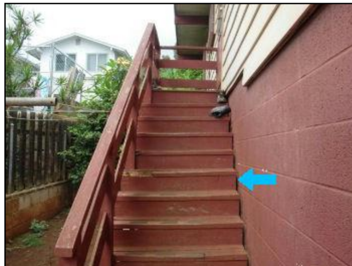
Steps or landings settling or heaving
