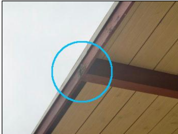
Rot or insect damage
