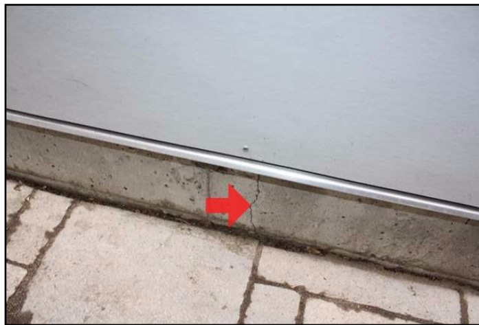
Example of typical minor crack
