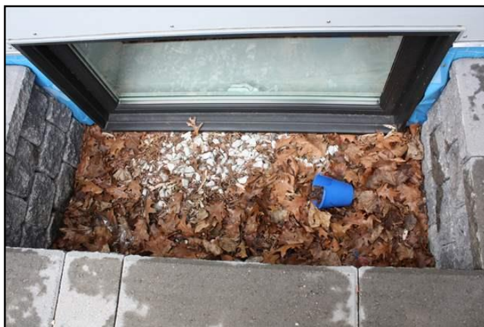
Window Well - missing 6 to 8 inches...
