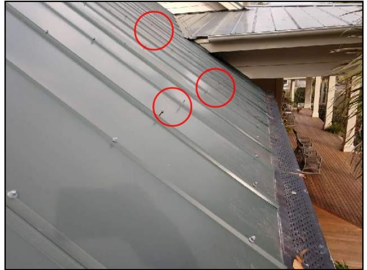
2. Failed fasteners
