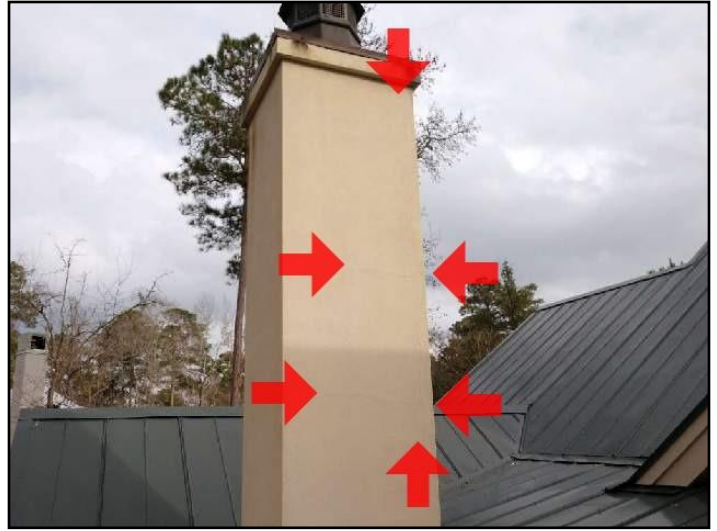
4. Cracks in stucco
