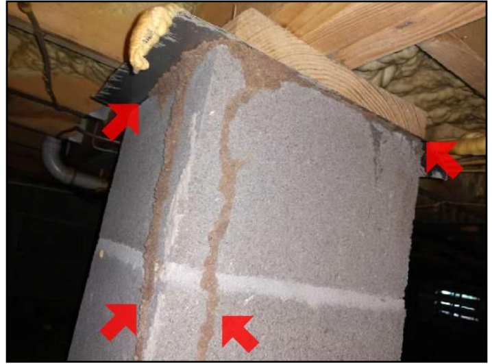
44. Evidence of wood destroying insects
