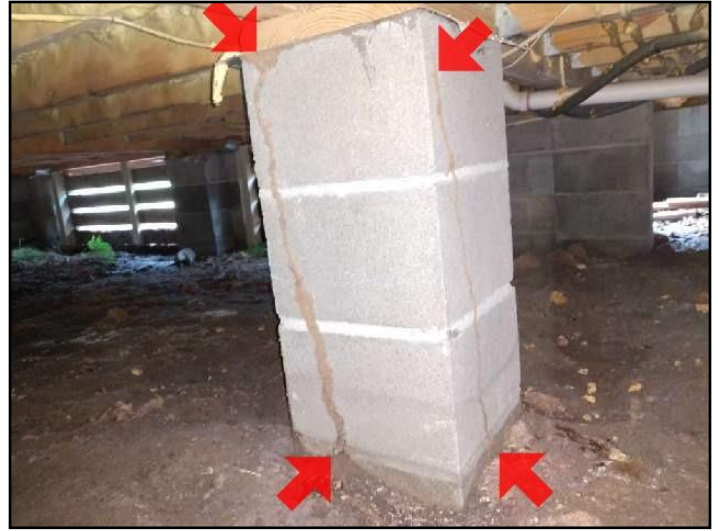
13. Evidence of wood destroying insects
