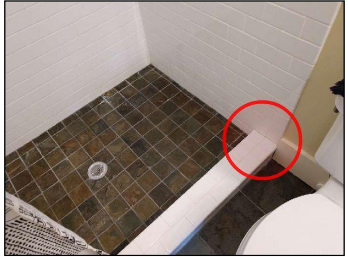
21. Grout loose, missing or deteriorated
