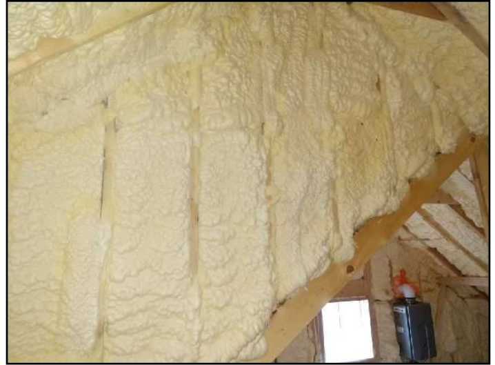
84. foam wall insulation
