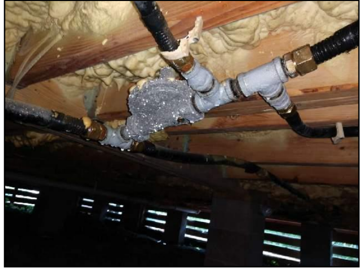
97. CSST (Corrugated Stainless Steel Tubing)
