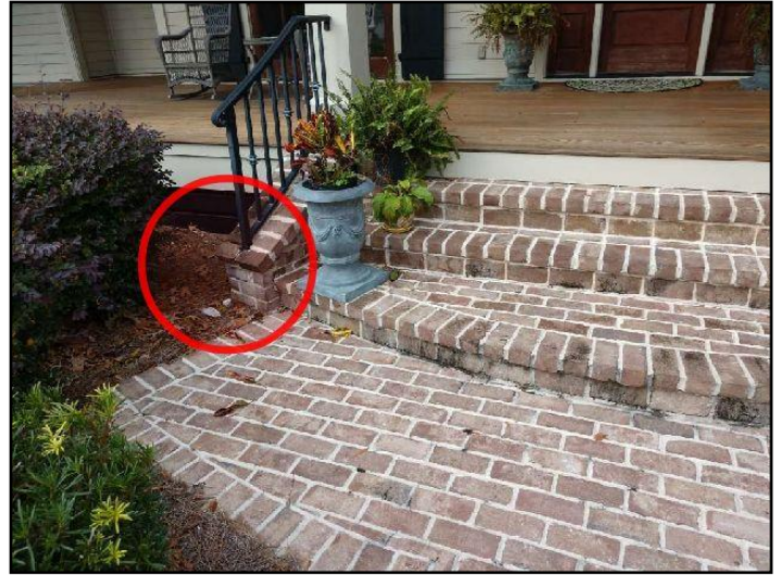
7. Masonry or concrete cracking
