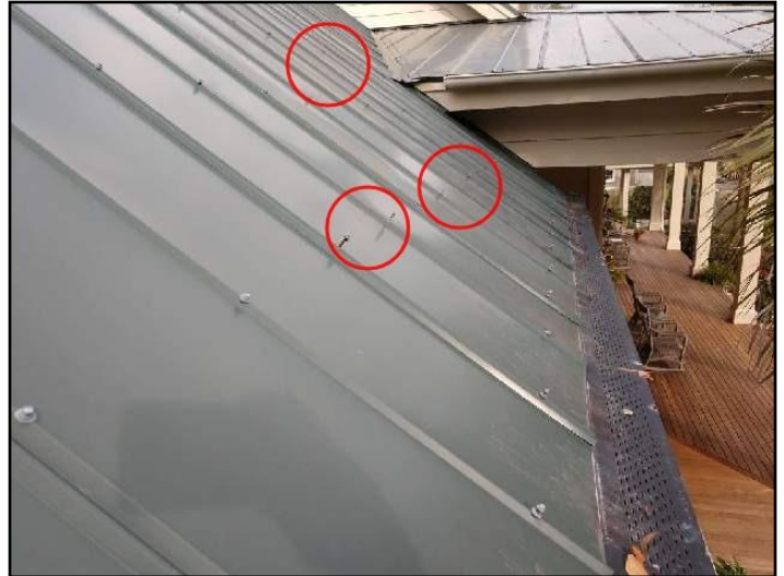
25. Failed fasteners
