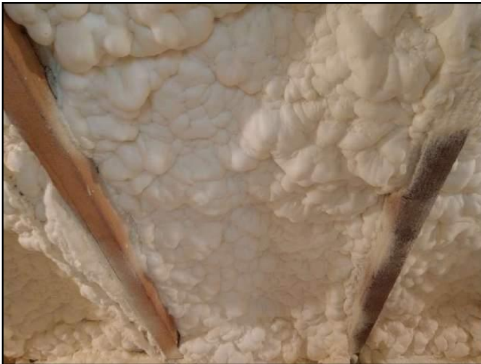
85. Foam floor insulation
