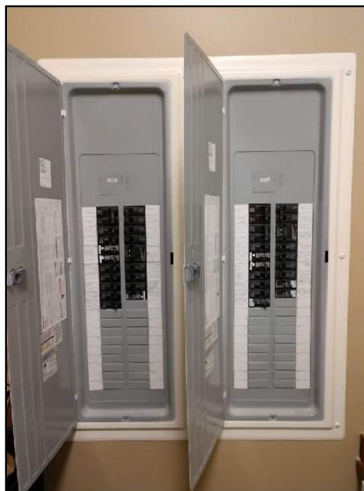
65. Siemens distribution panels (Laundry room)
