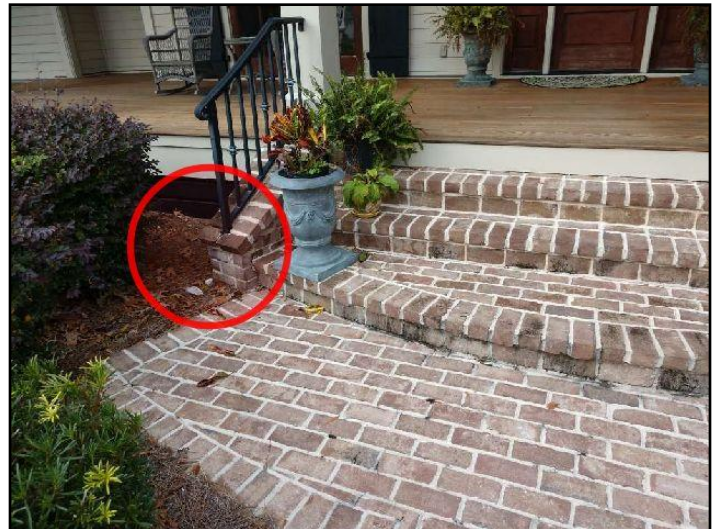
34. Masonry or concrete cracking
