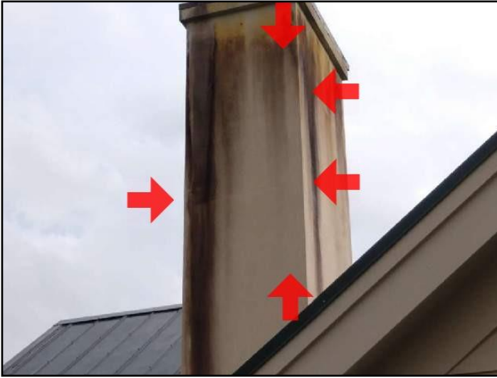
3. Cracks in stucco
