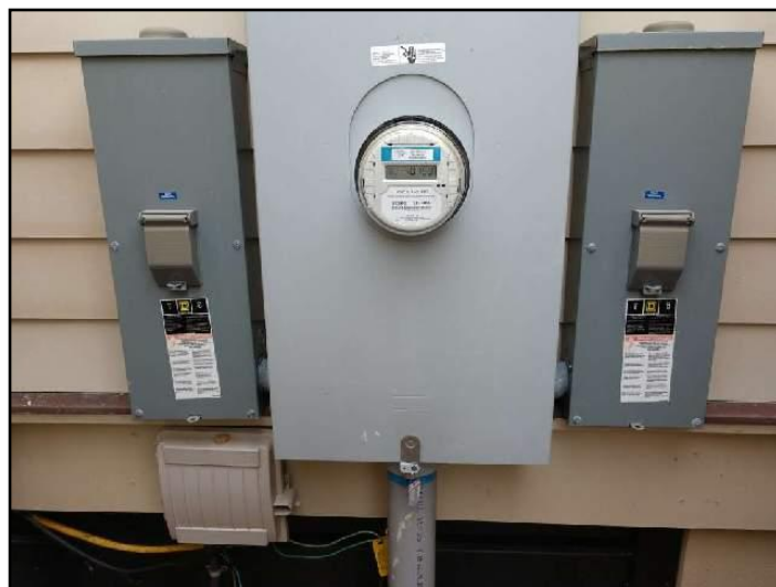
63. Square D main panels (Left exterior)
