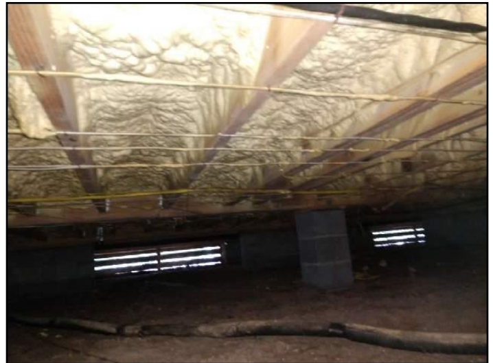
86. Foam floor insulation
