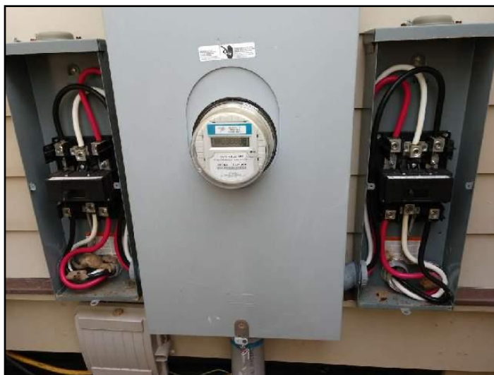
59. Underground, aluminum service entrance cable
