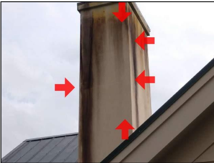
30. Cracks in stucco
