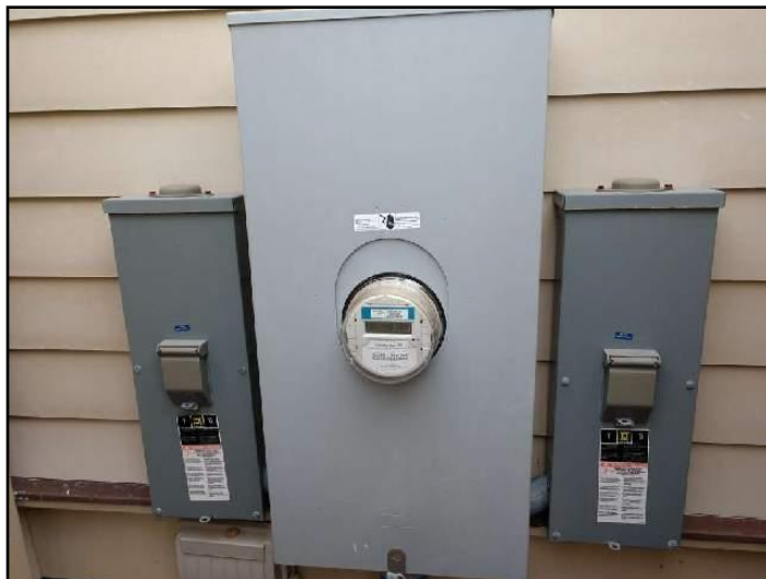
58. Service enters at the meter (Left exterior)
