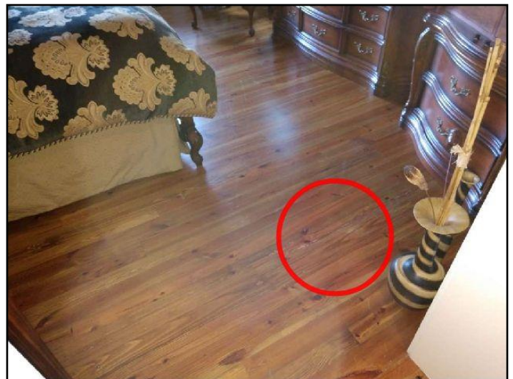
23. Insect damage to Floor boards
