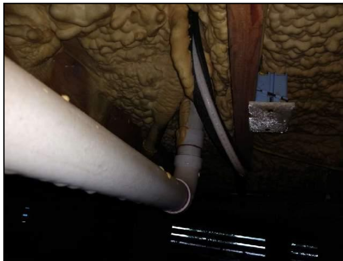
89. Foam obstruction - crawlspace
