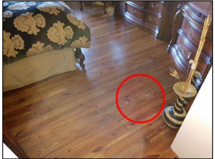
104. Insect damage to Floor boards
