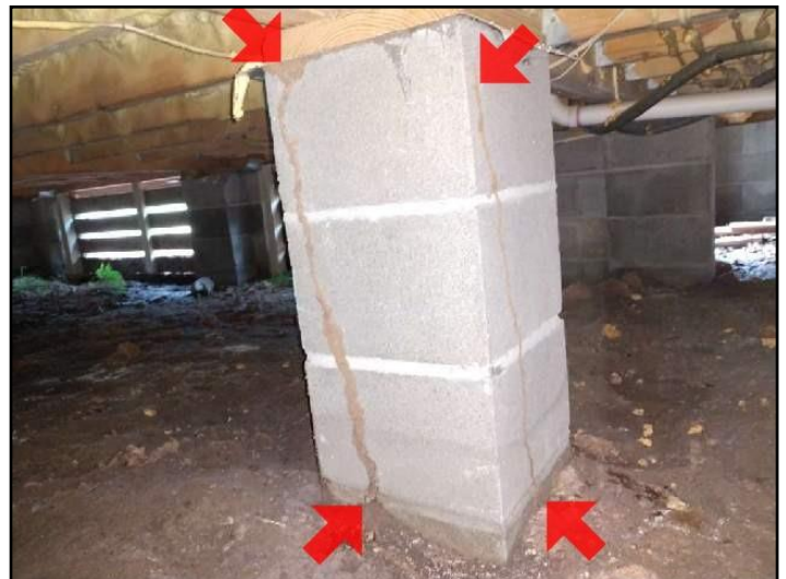
42. Evidence of wood destroying insects
