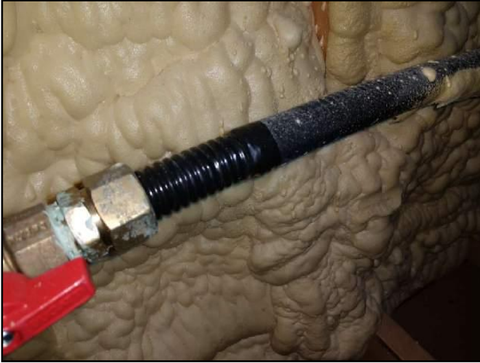
96. CSST (Corrugated Stainless Steel Tubing)
