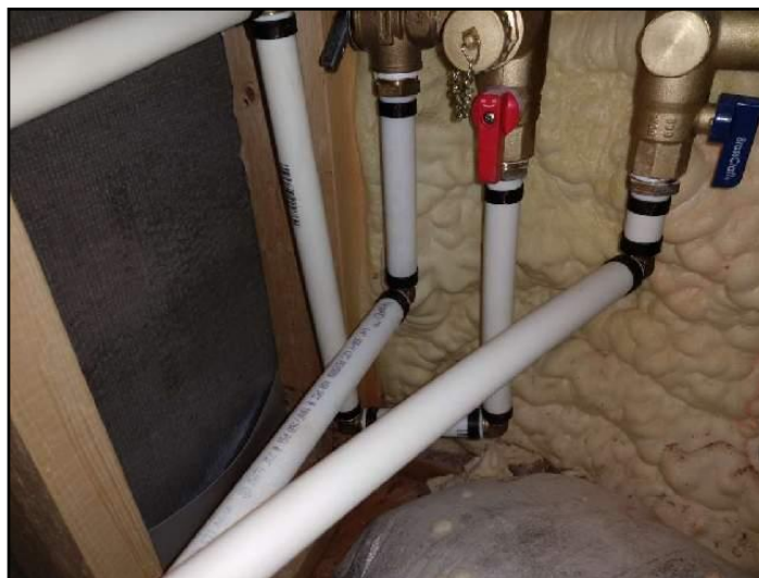
93. PEX (cross-linked Polyethylene)
