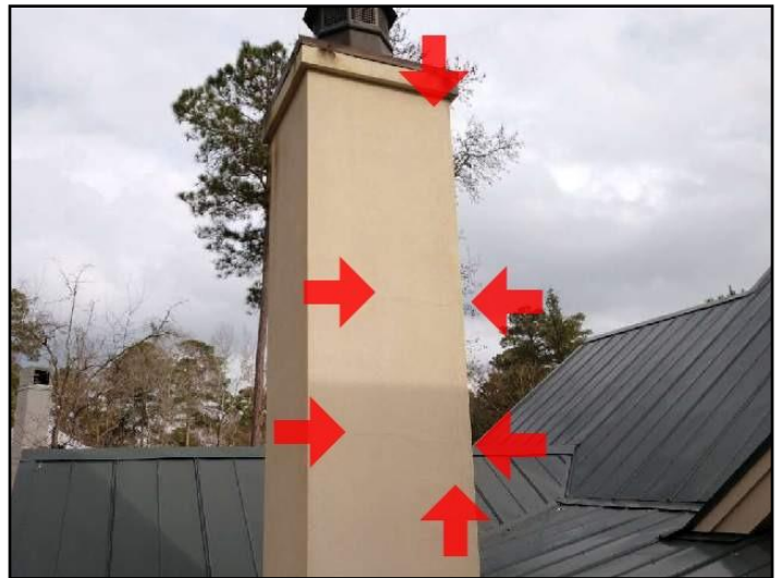
31. Cracks in stucco
