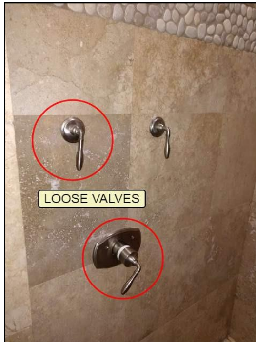
90. Valves are loose on the shower wall
