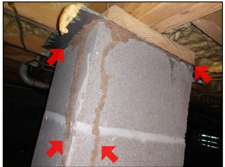
15. Evidence of wood destroying insects
