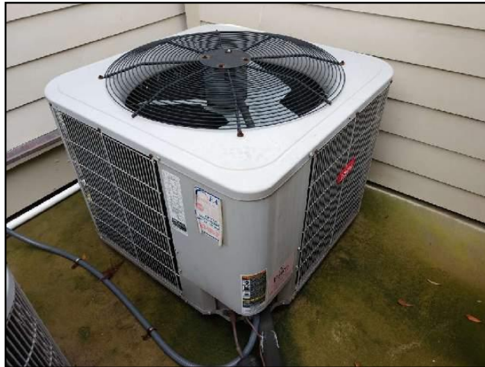
77. Exterior condensing unit, Main system
