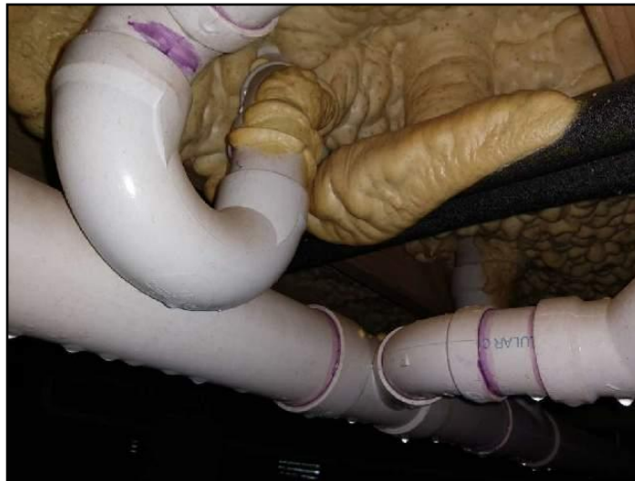
56. Foam insulation-obstruction
