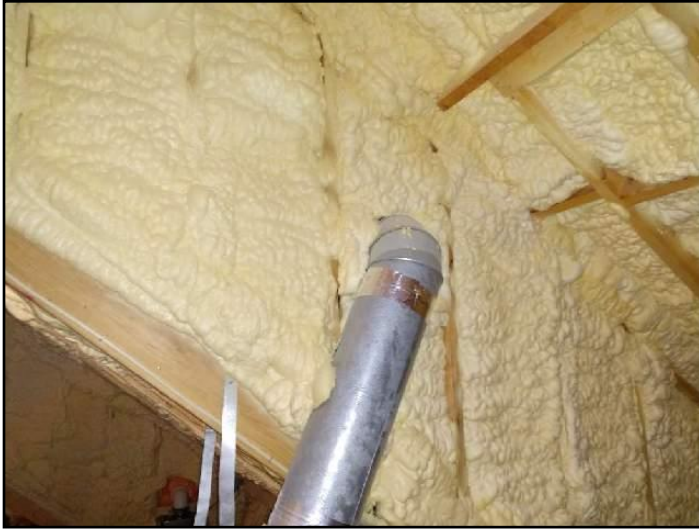
83. foam wall insulation
