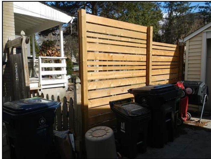
Spindles (balusters) climbable
