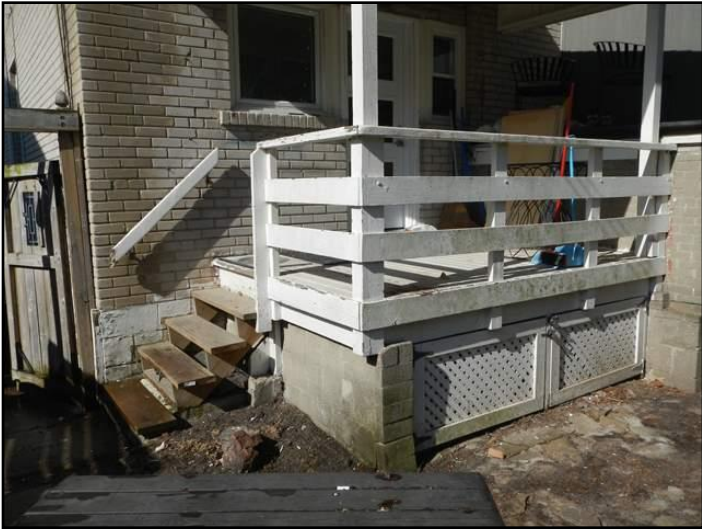
Spindles (balusters) climbable
