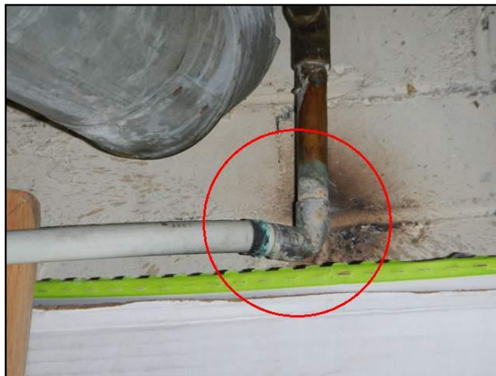
Corrosion
