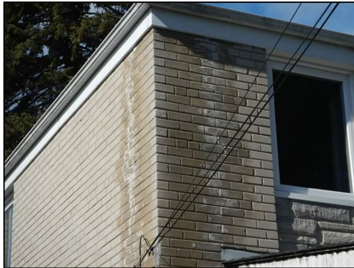
Efflorescence
