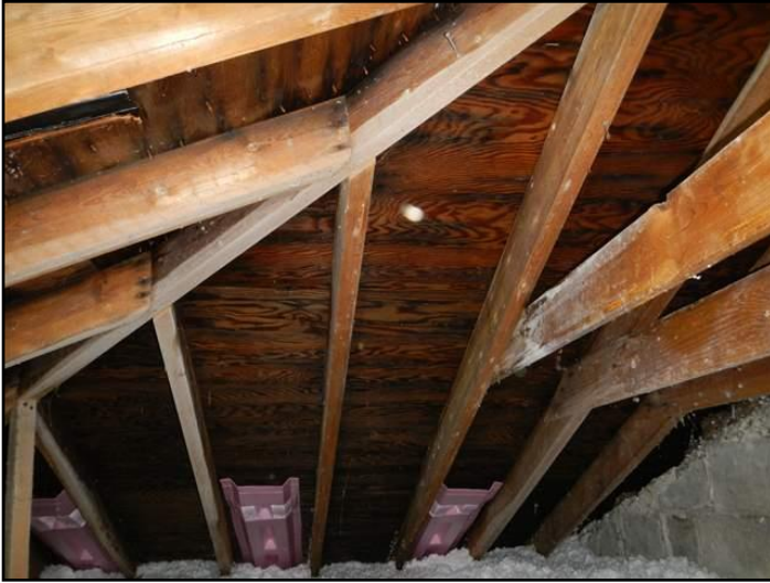
Rafters/roof joists
