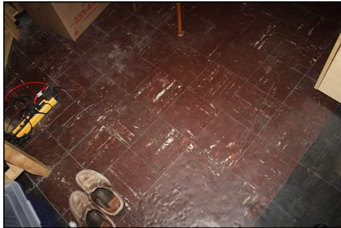
8. Possible asbestos containing materials
