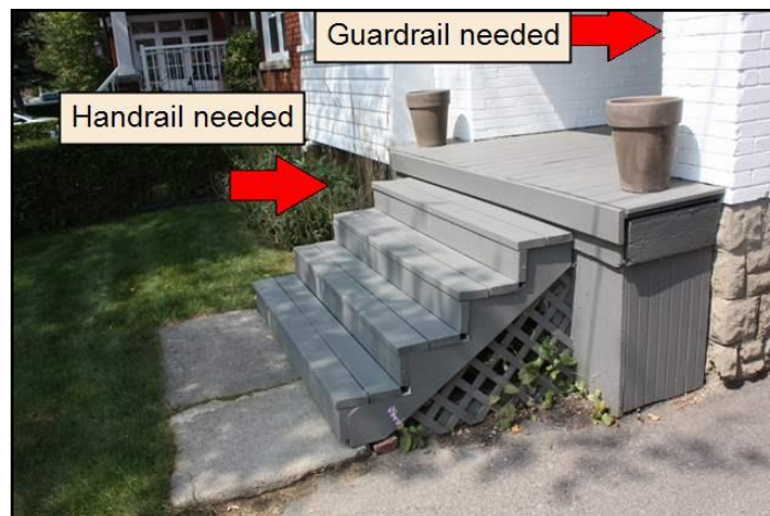
7. Missing Hand and Guardrail
