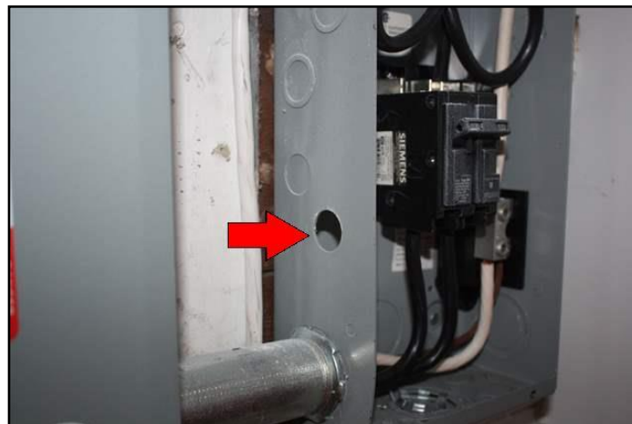
14. Unprotected openings
