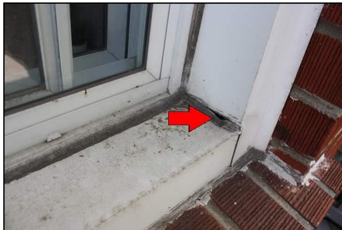
4. Caulking missing or ineffective
