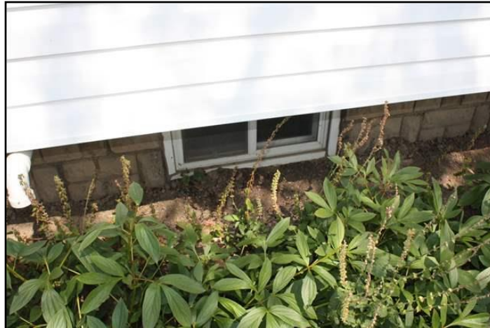
5. Sill - Near or at Grade Level
