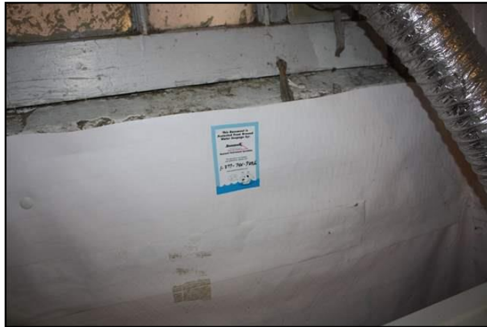
26. New dampproofing material
