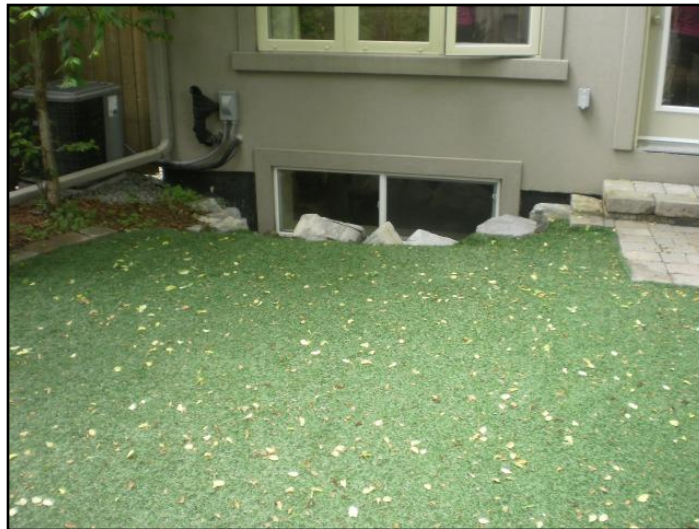
12. Improper slope
