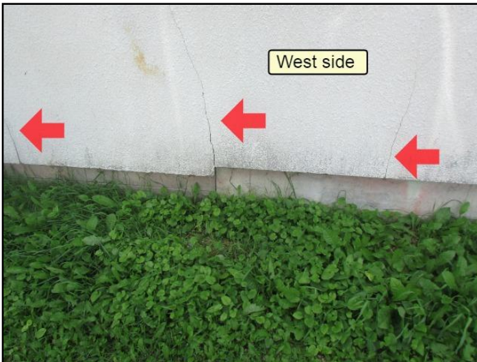
16. Typical minor cracks
