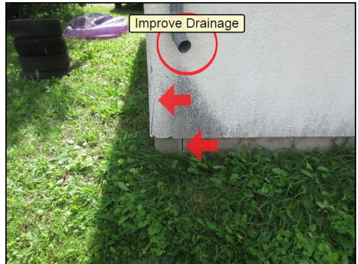
17. Typical minor cracks
