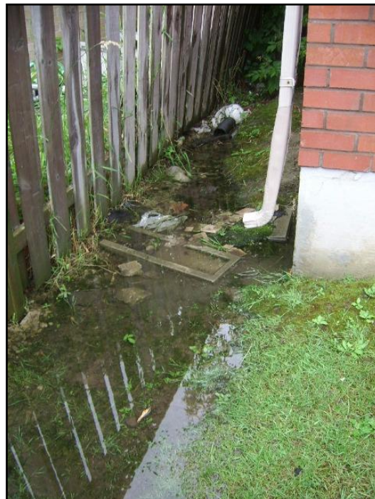
10. Downspouts end too close to building
