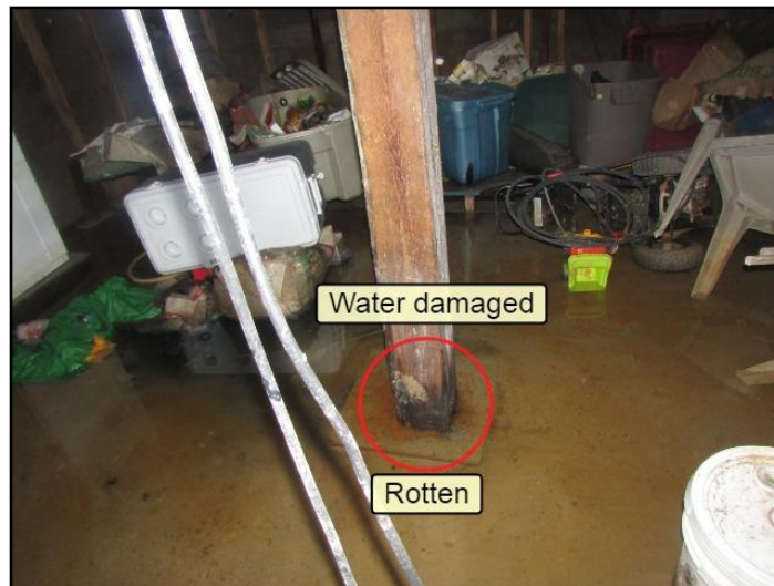
19. Rot or insect damage
