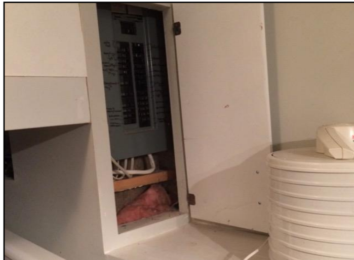
Box location poor
