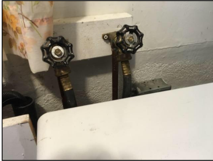
rubber supply line, prone to fail
