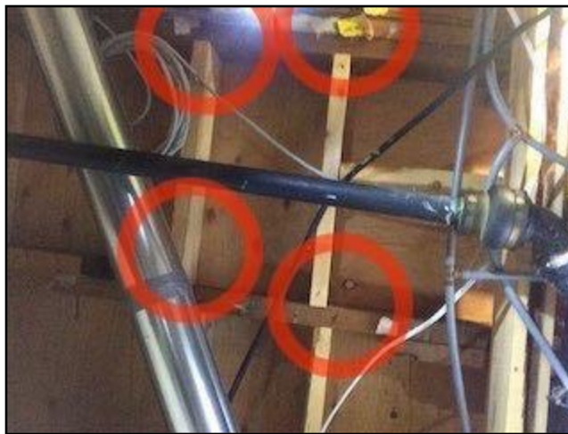
Ineffective blocking, bracing or bridging
