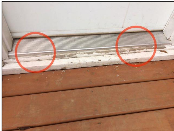
Paint and Caulking - deteriorated / missing
