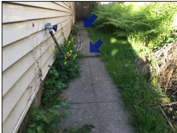
Improper slope
