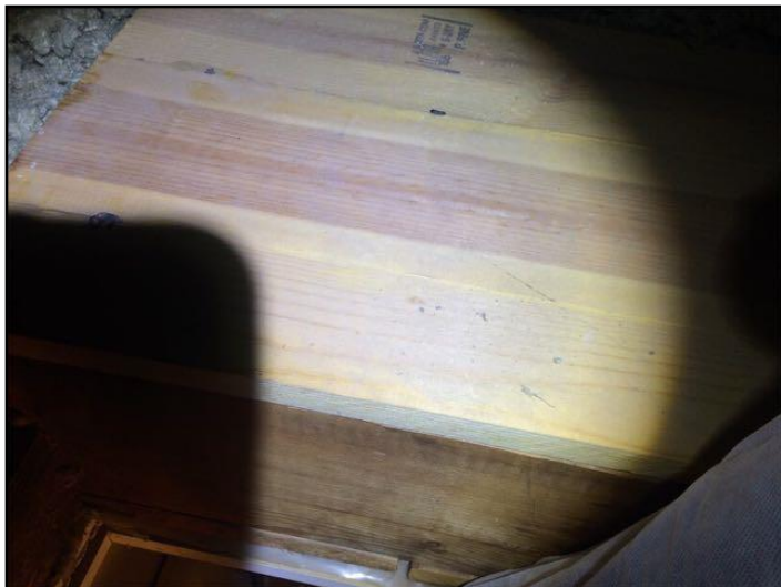
Not insulated and not weatherstripped
