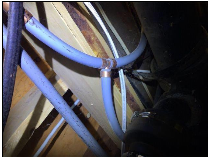
Suspect polybutylene connections
